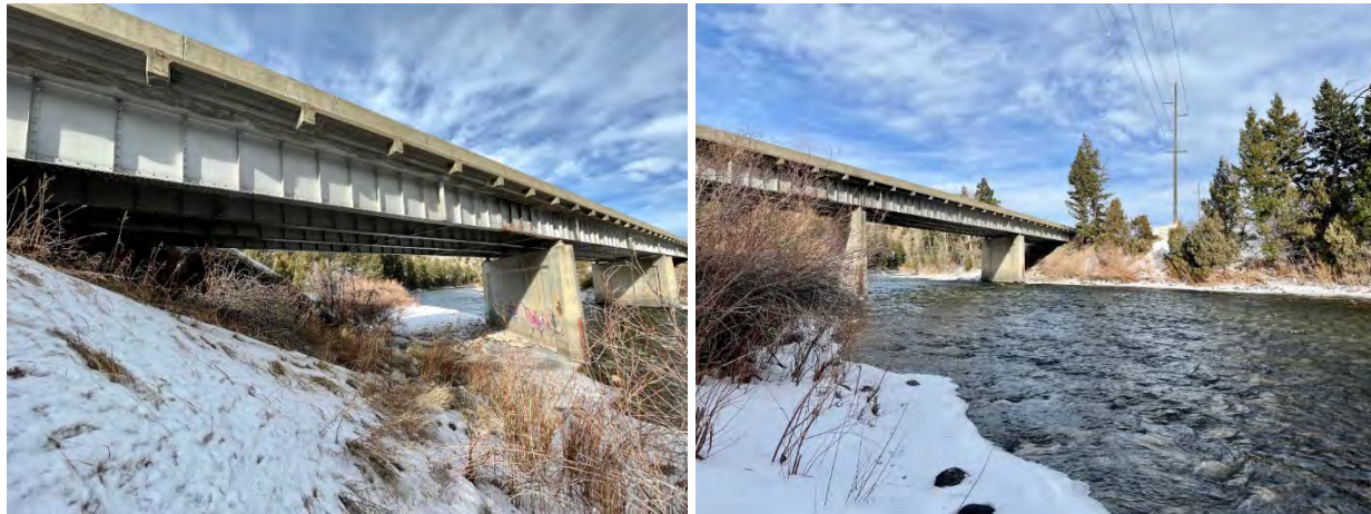
Figure 27 Gallatin River Bridge (RM 70.5)
