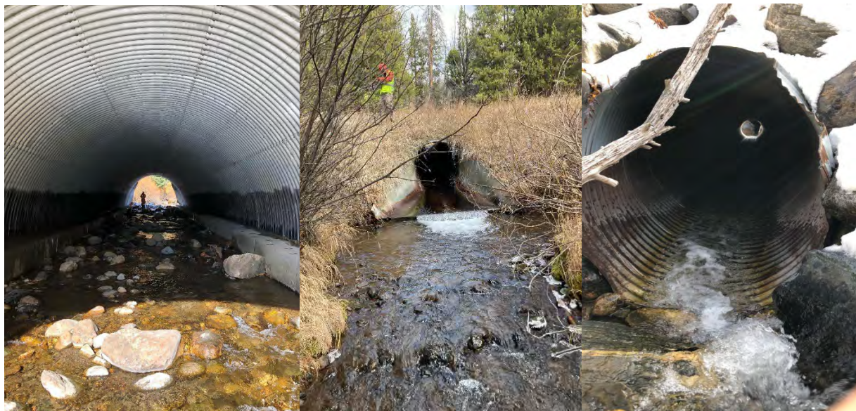
Figure 42 Aquatic Passage Assessment: Images of a “Green” Crossing (left), a “Gray” Crossing (middle), and a “Red” Crossing (right)
