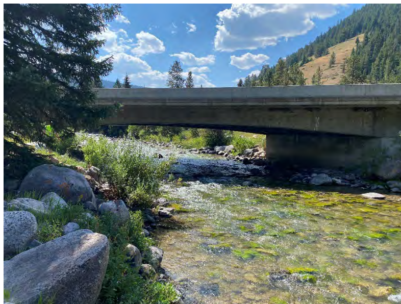
Figure 22 Bridge over Taylor Fork (RM 33.9)
