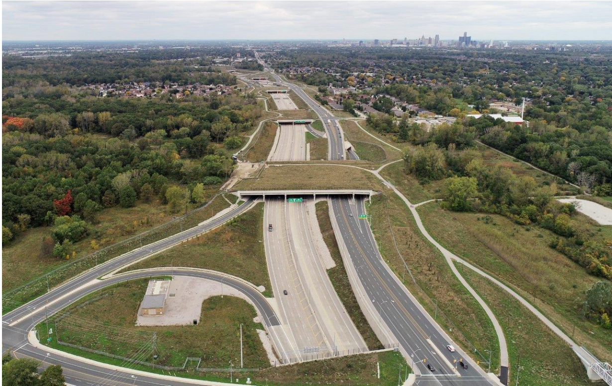
Figure 13: Aerial imagery of a wildlife overpass for snakes in Ontario showing bike path and the vegetation on top of the overpass connecting the habitat on the two sides of the highway. Photo Credit: Ministry of Transportation Ontario, Wood Environment & Infrastructure Solutions.
