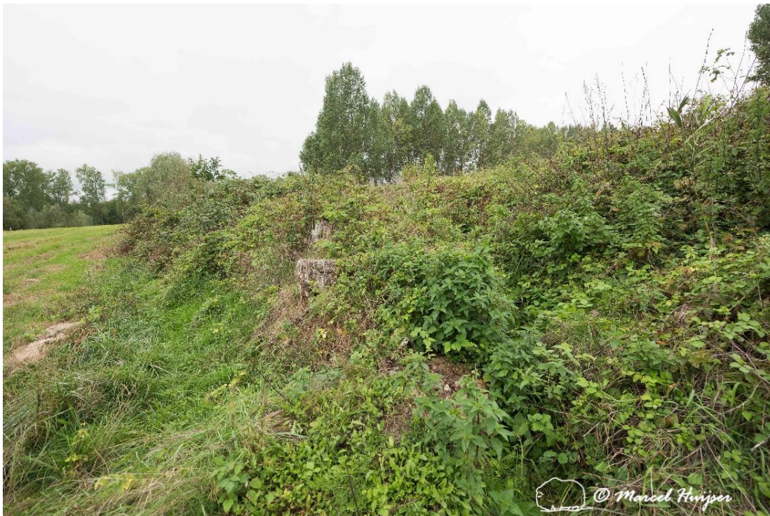
Figure 12: Detail of the berm in the dry zone. It consists of soil, root wads, shrubs (including thorny species such as bramble ( Rubus spp.)).
