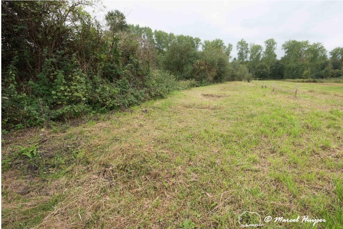
Figure 11: The wet zone is protected from cattle (used as a tool in nature management in the area) with a livestock fence (fence is on right side in the image). Note the small dams just above the center of the image that result in small pools during wetter times of the year. One of the berms is on the left side, at one of the outer edges of the overpass.
