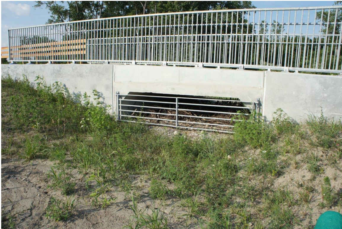
Figure 15: Detail of the underpass for snakes under a bicycle path on top of the wildlife overpass in Windsor, Ontario. Photo Credit: Ministry of Transportation Ontario, Wood Environment & Infrastructure Solutions.
