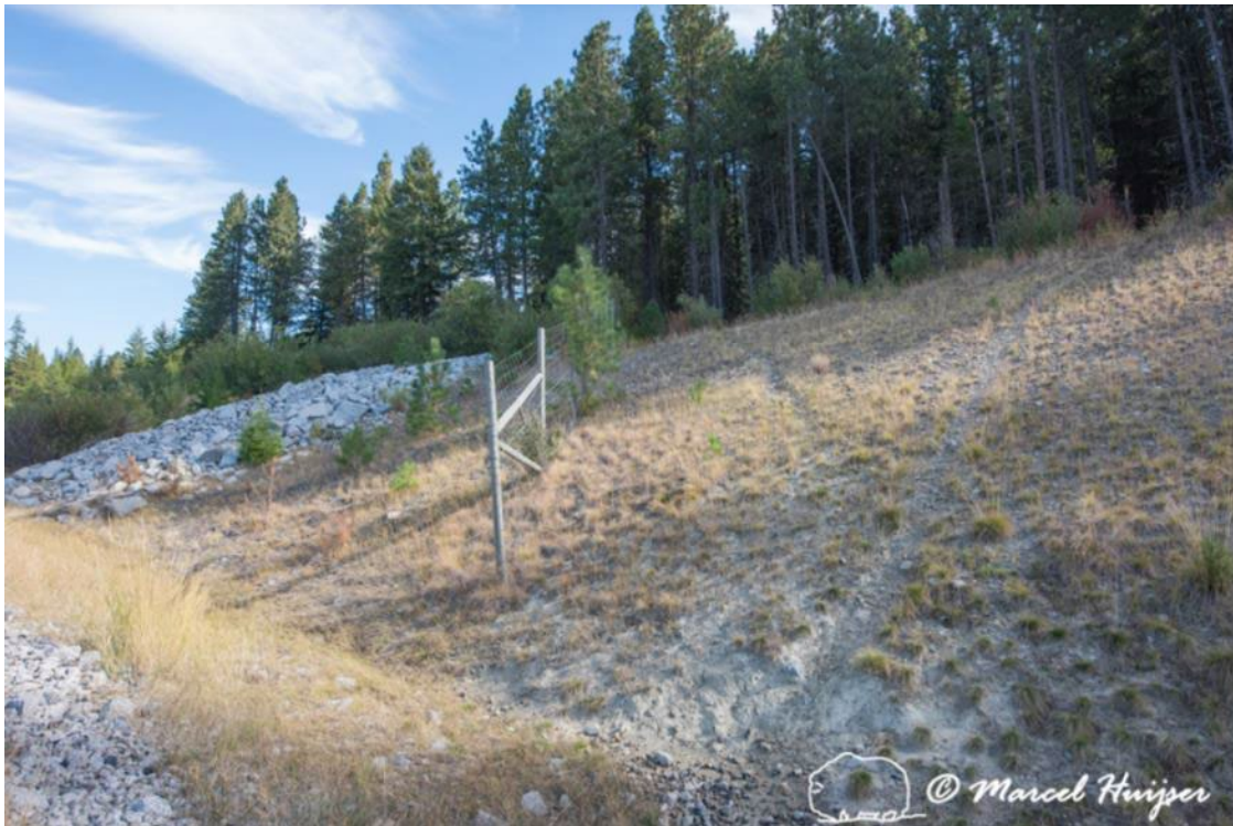
Figure 42. Wildlife trail at a fence-end, US Hwy 95, Bonners Ferry, Idaho, USA. This is an indication that there is a concentration of wildlife crossings at the fence-end (a “fence-end run”), potentially resulting in a concentration of collisions at or near the fence-end, just inside or just outside the fenced road section.
