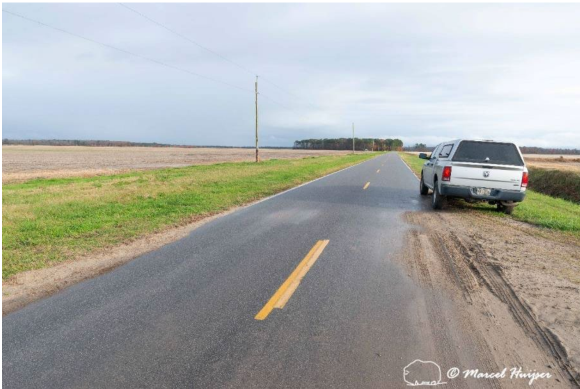
Figure 73: Frying Pan Rd., North Carolina.
