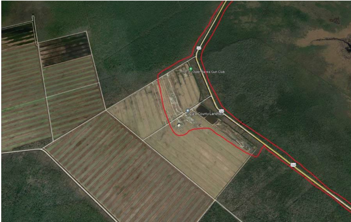
Figure 63: US Hwy 264, suggested wildlife fence around the landfill and gun club, Alligator River NWR, North Carolina.
