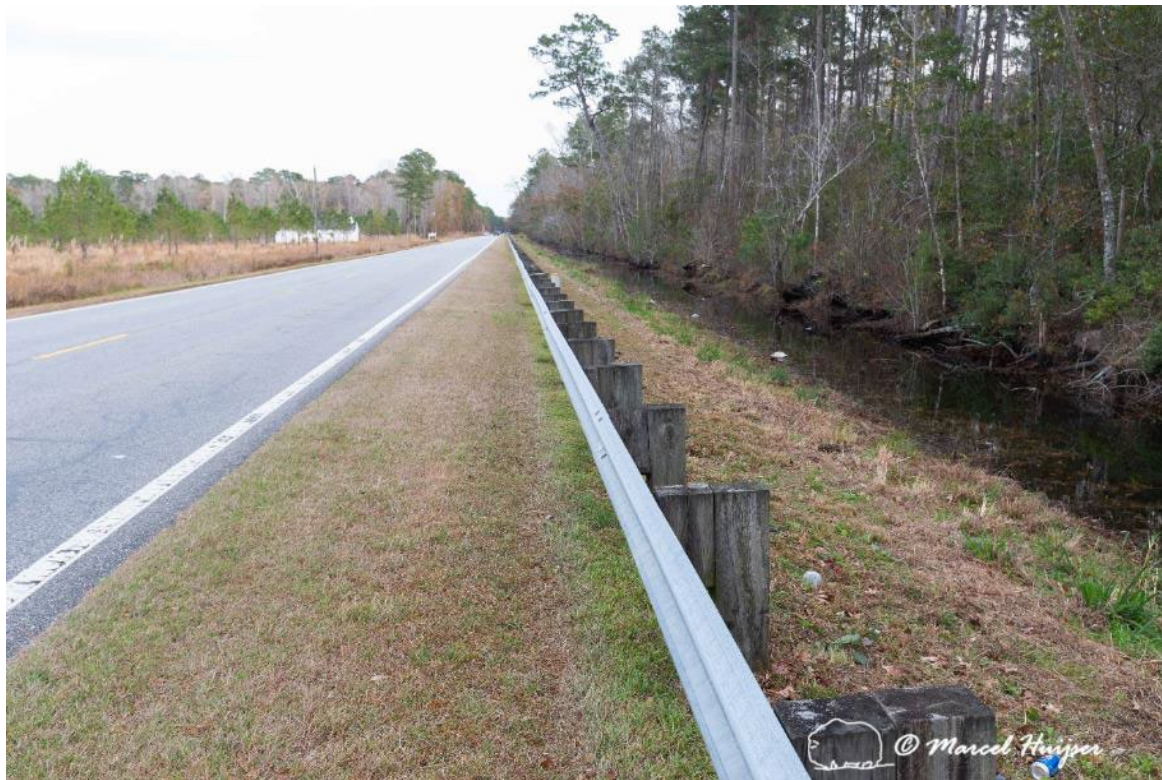
Figure 56: US Hwy 64, near Lake Neighborhood Rd, North Carolina.
