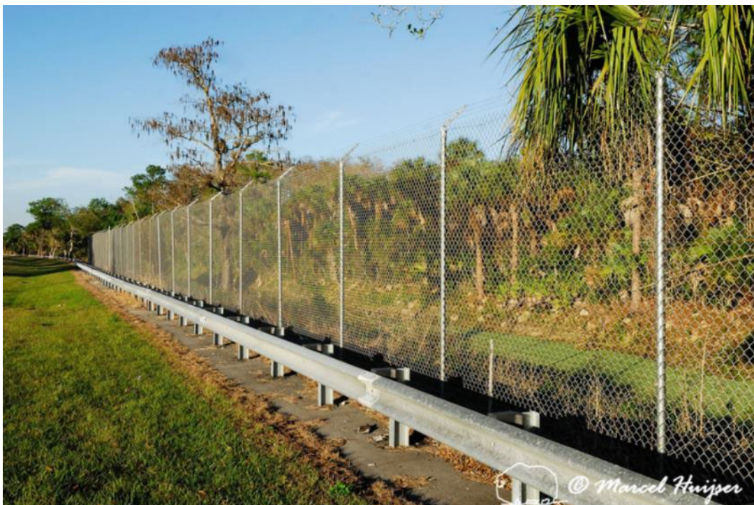
Figure 36. Fence for Florida panther ( Puma concolor coryi ), 10 ft tall, metal posts, chain-link fence material, and overhang or outrigger, SR 29, Florida, USA).
