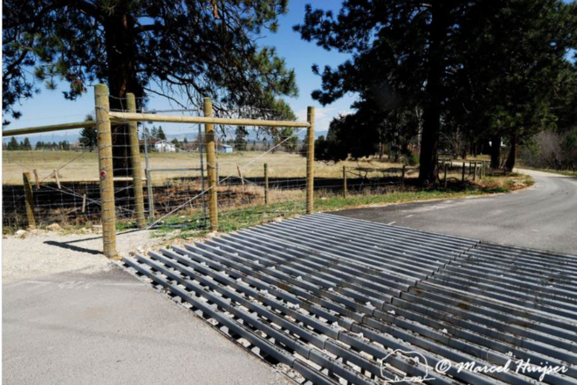
Figure 45. Wildlife guard at an access road to US Hwy 93S, near Victor, Montana, USA. This type of wildlife guard is less suited for pedestrians and cyclists.
