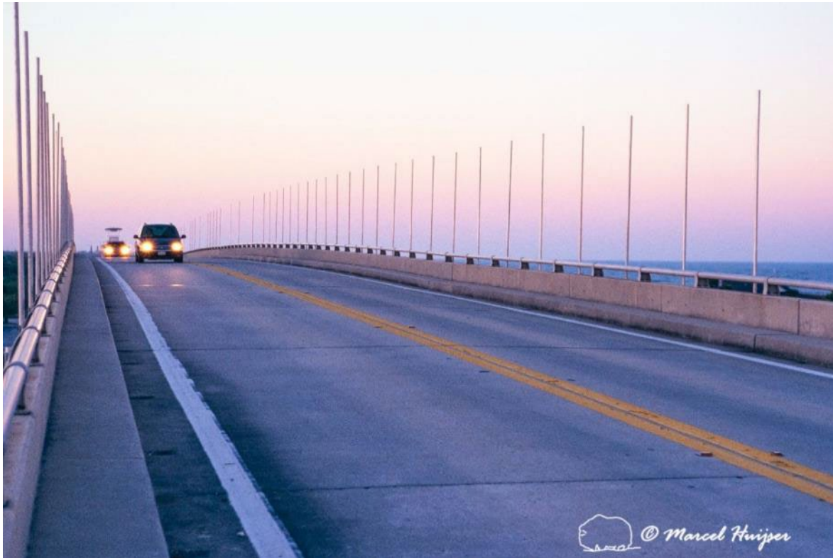
Figure 50: Metal poles attached to bridge to reduce bird-vehicle collisions by making the birds fly higher, State Road A1A, Sebastian Inlet State Park, Florida.
