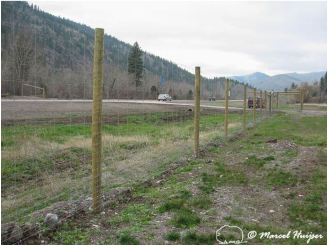
Figure 35. Typical large ungulate fence in North America, 8 ft tall, wooden posts and mesh-wire fence material, US Hwy 93 North, Montana, USA. Note that there is a dig barrier attached to the main fence material (e.g., for canids).
