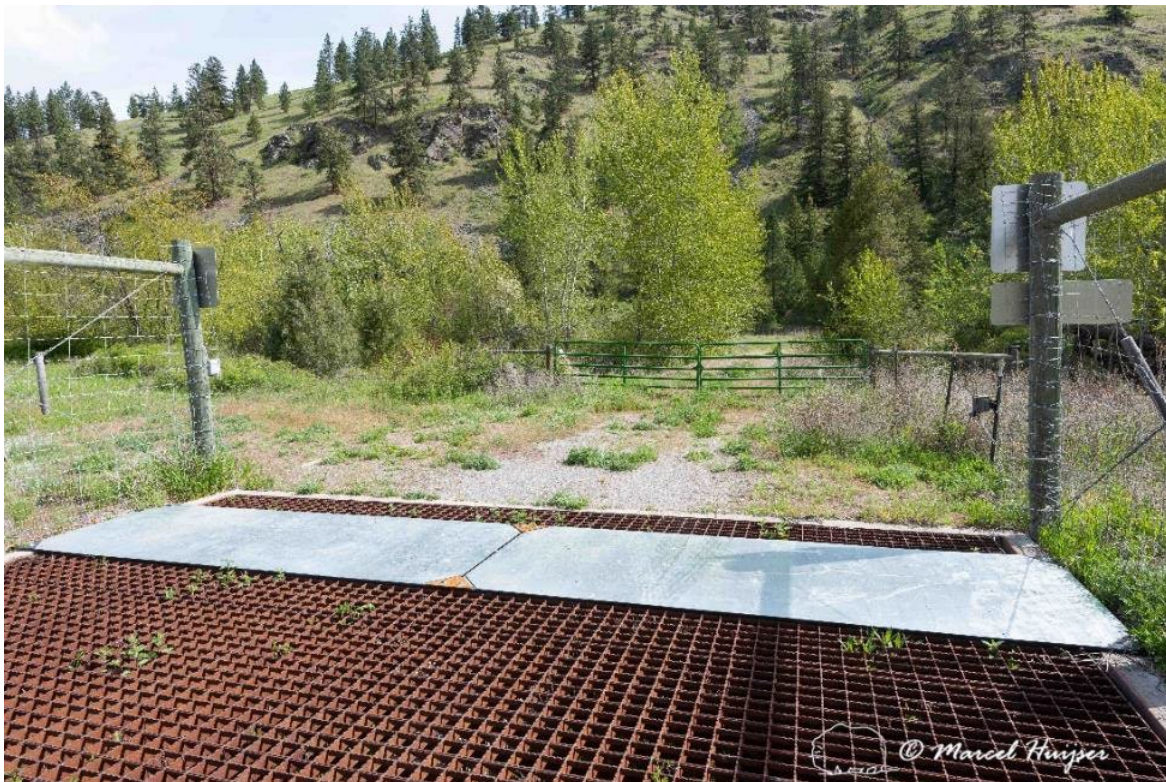
Figure 46. Electrified barrier, designed for low traffic volume and low traffic speed, on top of a wildlife guard at an access road to US Hwy 93S, near Ravalli, Montana, USA.
