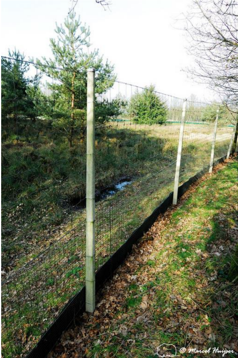
Figure 51. Wildlife fence for amphibians (e.g., common toad ( Bufo bufo )), medium sized mammals (e.g., Eurasian badger ( meles meles )) and large ungulates (e.g., roe deer ( Capreolus capreolus ), red deer ( Cervus elaphus )) at ecoduct Woeste Hoeve A50 near Apeldoorn, The Netherlands.
