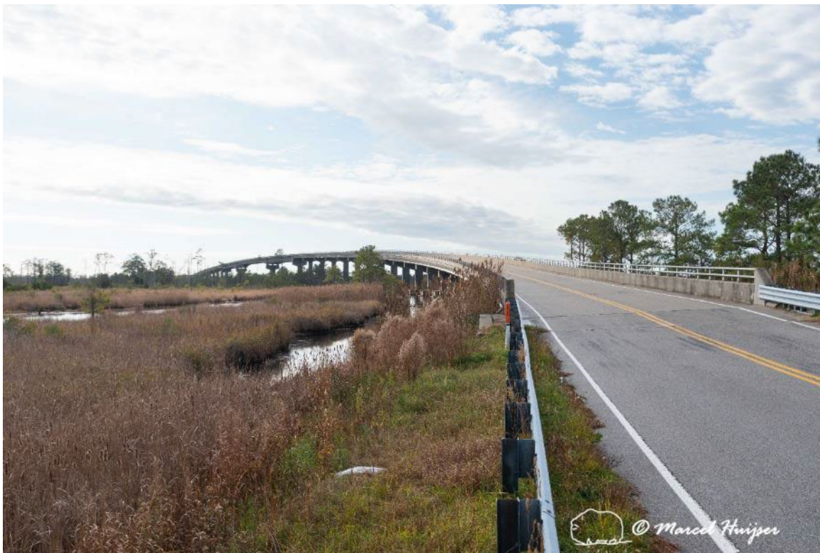
Figure 77: Hwy 94, bridge across Intracoastal Waterway, north of Fairfield, North Carolina.
