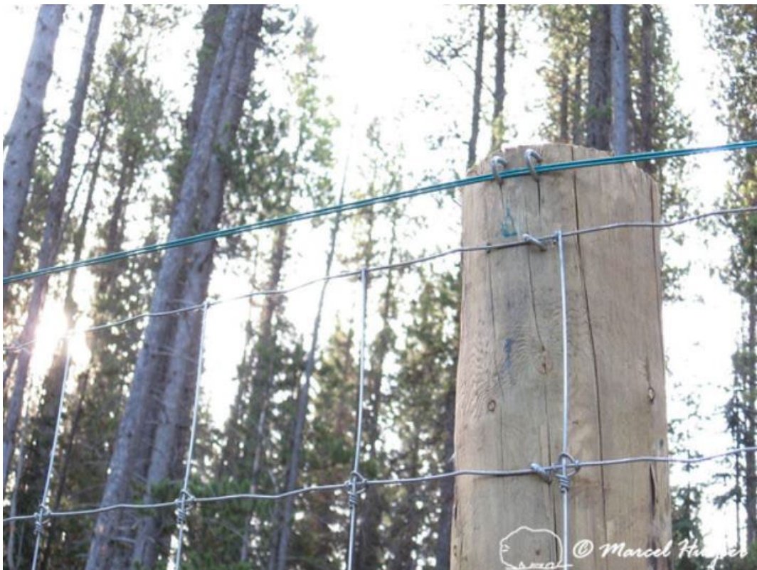
Figure 40: Wildlife fence with high-tensile top wire to reduce damage from falling trees, Trans-Canada Highway, Banff National Park, Alberta, Canada.
