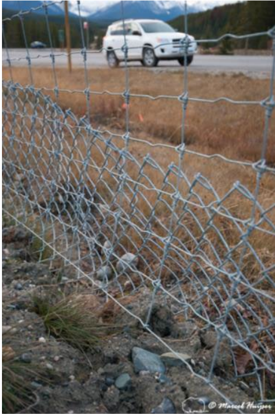
Figure 37. Wildlife fence and dig barrier (“buried fence” or “apron”), Trans-Canada Highway, Banff National Park, Alberta, Canada. The dig barrier in the soil angles (45°) towards the safe side or habitat side; it angles away from the fence and the road on the other side (Clevenger and Huijser 2011). The dig barrier keeps animals from digging under the fence. The dig barrier may consist of a 4-5 ft (1.0-1.2 m) wide galvanized chain-link fence that is attached to the bottom of the actual fence. The buried fence should extend approximately 3.5 ft (1.1 m) under the ground (Clevenger and Huijser 2011).
