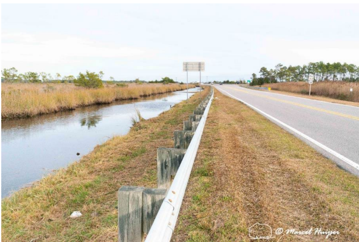
Figure 59: US Hwy 64 and adjacent canal, just west of the junction with US Hwy 264, Alligator River National Wildlife Refuge, North Carolina.
