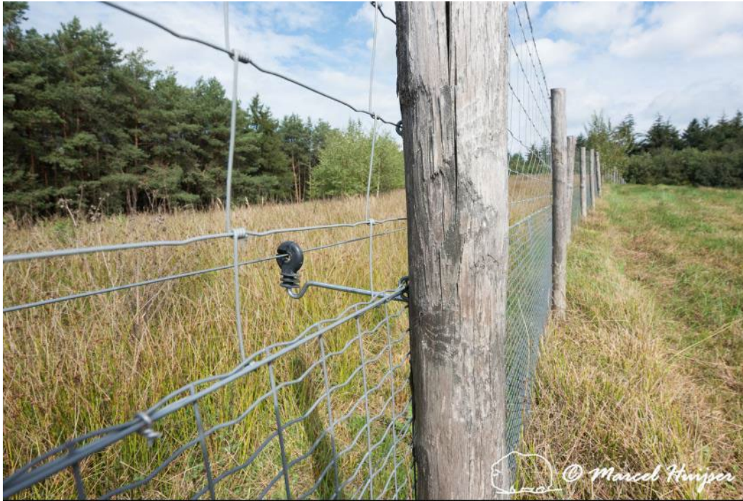
Figure 39: Wildlife fence along A28 motorway, near Spier, Drenthe, The Netherlands. The fence is a barrier for medium and large mammal species. The electrified wire is an additional barrier to keep animals out of the fenced road corridor.
