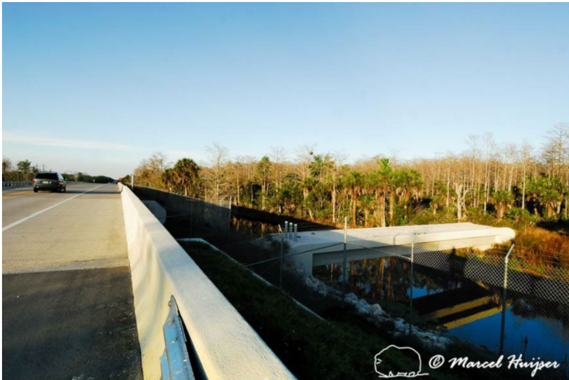
Figure 53: Wildlife underpass for Florida panthers ( Puma concolor coryi ) (on the left, under the road), and a wildlife bridge across canal leading up to the underpass (on the right), SR 29, Florida, USA.
