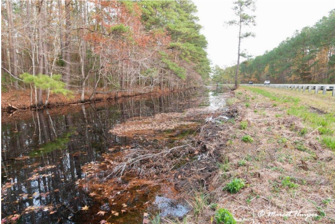
Figure 57: US Hwy 64 and adjacent canal at Buffalo City Rd., Alligator River National Wildlife Refuge, North Carolina.
