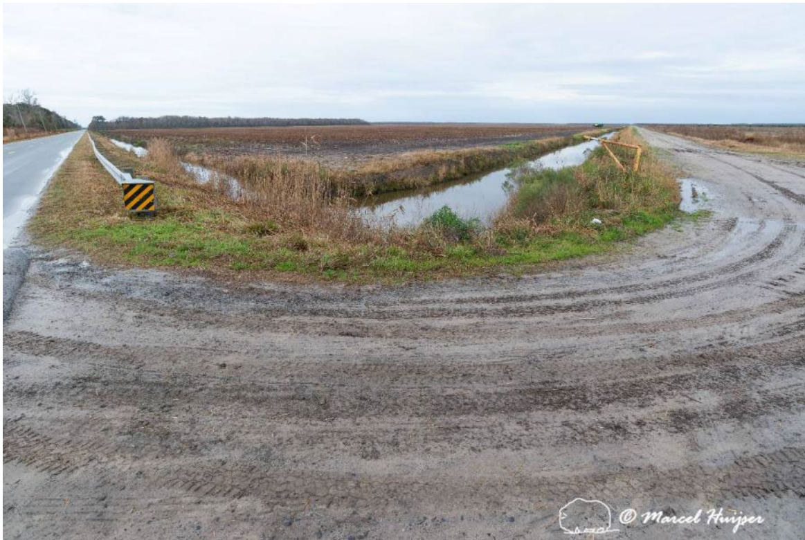
Figure 68: US Hwy 264, US Hwy 264, north of Engelhard at junction with Smith Ave, North Carolina.
