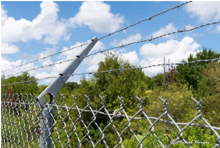
Figure 38. Outrigger or overhang on a fence for Florida panther ( Puma concolor coryi ), SR 29, Florida, USA. Note that the outrigger faces the safe side, the habitat side of the fence. A longer overhang from chain-link fence material is suggested for red wolf.
