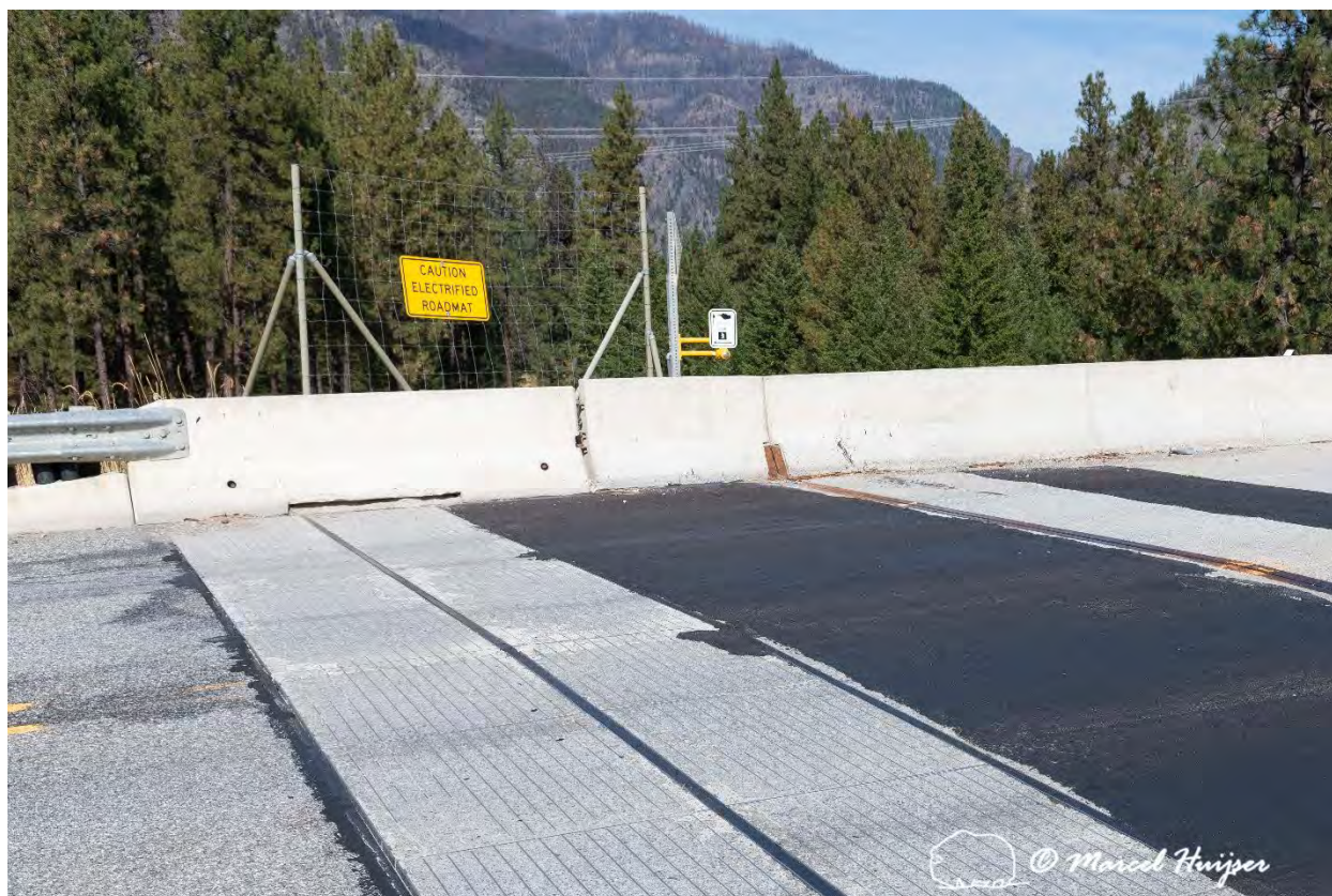
Figure 38: The crumbling concrete at the western electrified barrier was covered in asphalt.
