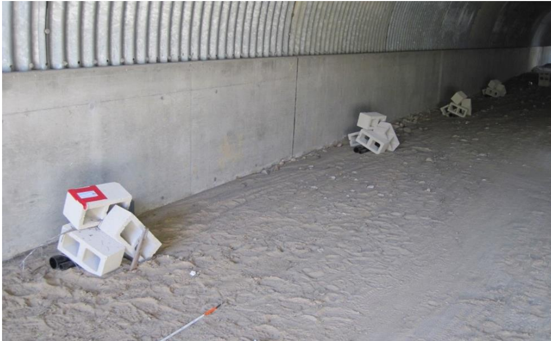
Figure 2: Cinder blocks laid on top of black PVC pipe in a dry culvert built for larger animals. Photo Credit: (For a U.S. Geological Survey project) Jeff Tracey, Western Ecological Research Center, U.S. Geological Survey.
