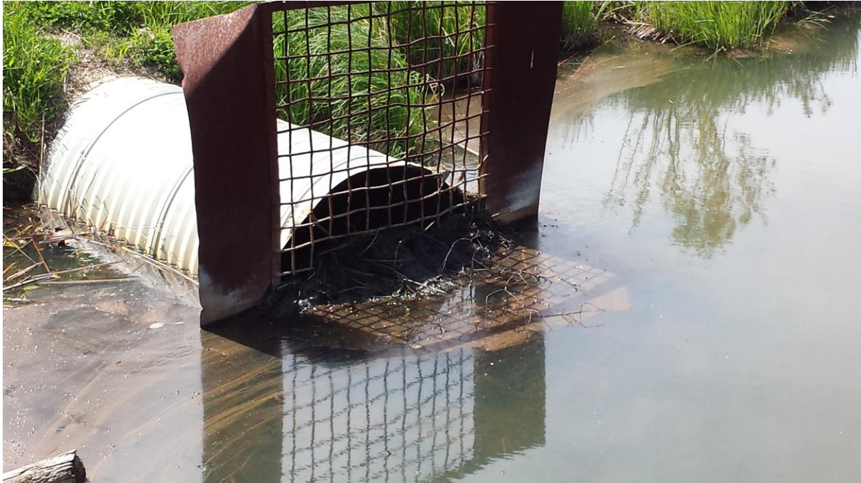
Figure 1: A metal grate on a drainage culvert to deter beaver access and associated beaver dams inside drainage culvert; these screens impede movement by turtles and other animals through drainage culvert. Photo Credit: Ausable Bayfield Conservation Authority.
