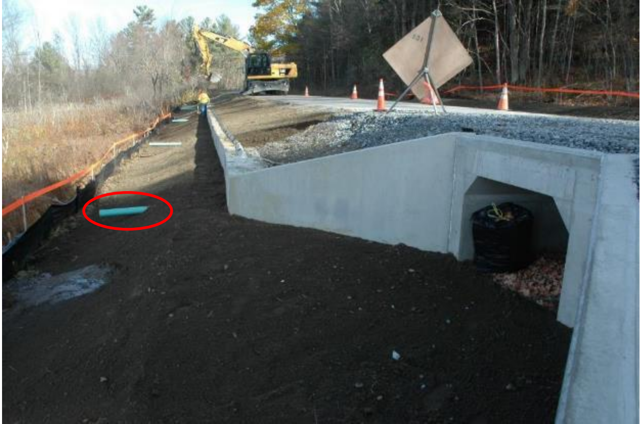
Figure 4: Concrete guide-walls used to funnel amphibians into the bottomless underpass and drainage pipes (red circle) inserted underneath the guide-wall. Photo Credit: Chris Slesar, Monkton Conservation Commission.
