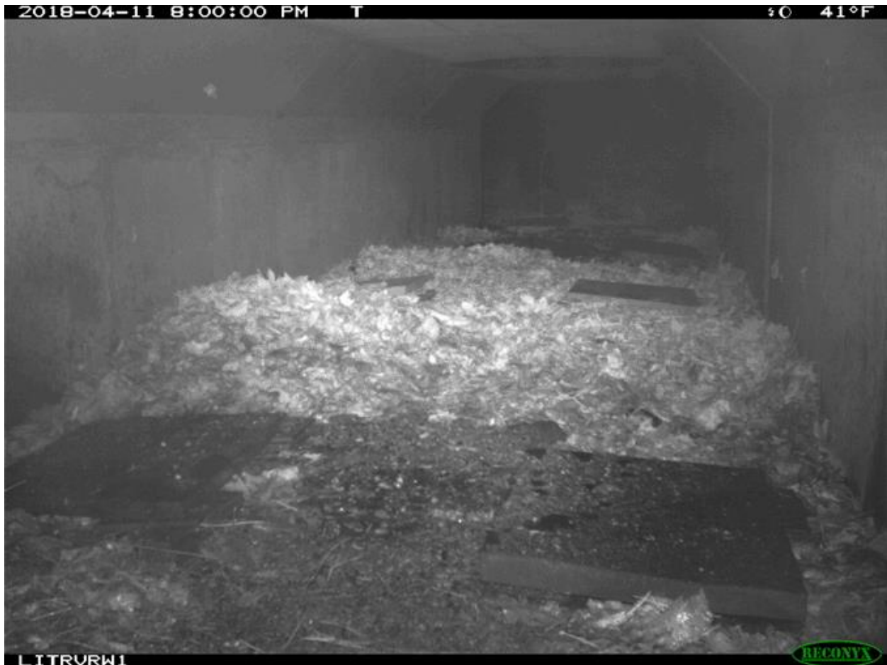
Figure 8: Figure shows the inside of the underpass with cover objects; it is actually a video (.gif) that shows amphibians moving through. Video Credit: Chris Slesar, Monkton Conservation Commission.
