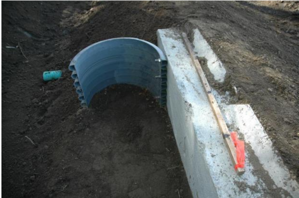
Figure 5: Plastic corrugated HDPE pipe used at barrier end to redirect amphibians away from the road. Photo Credit: Chris Slesar, Monkton Conservation Commission.
