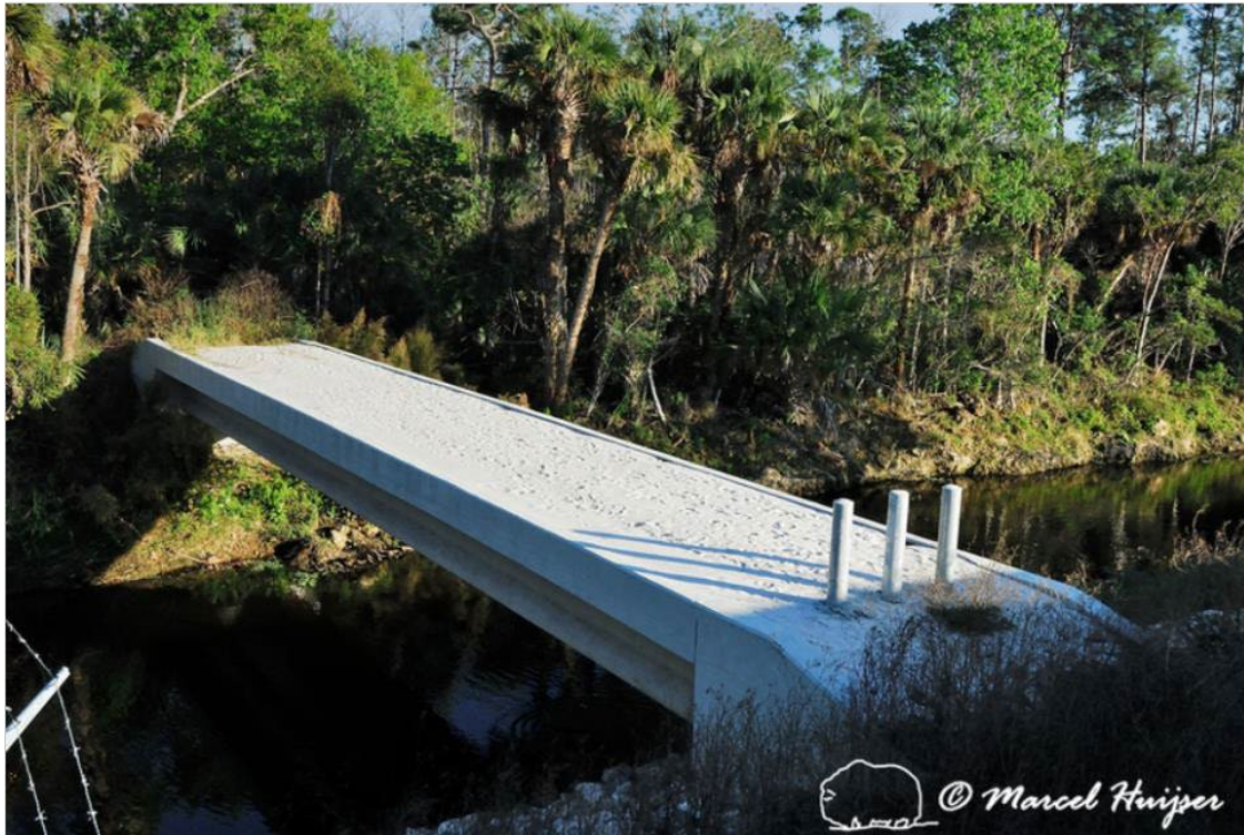
Figure 54: Wildlife underpass for Florida panthers ( Puma concolor coryi ) (to the right, outside of image) and a wildlife bridge across canal, SR 29, Florida, USA. Note that the posts on the bridge block illegal use of motorized vehicles such as ATVs.
