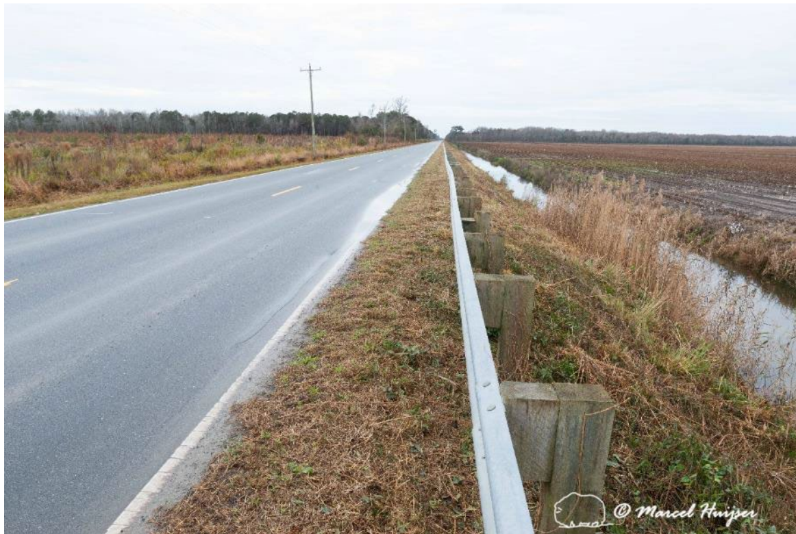
Figure 69: US Hwy 264, north of Engelhard at junction with Smith Ave, North Carolina.
