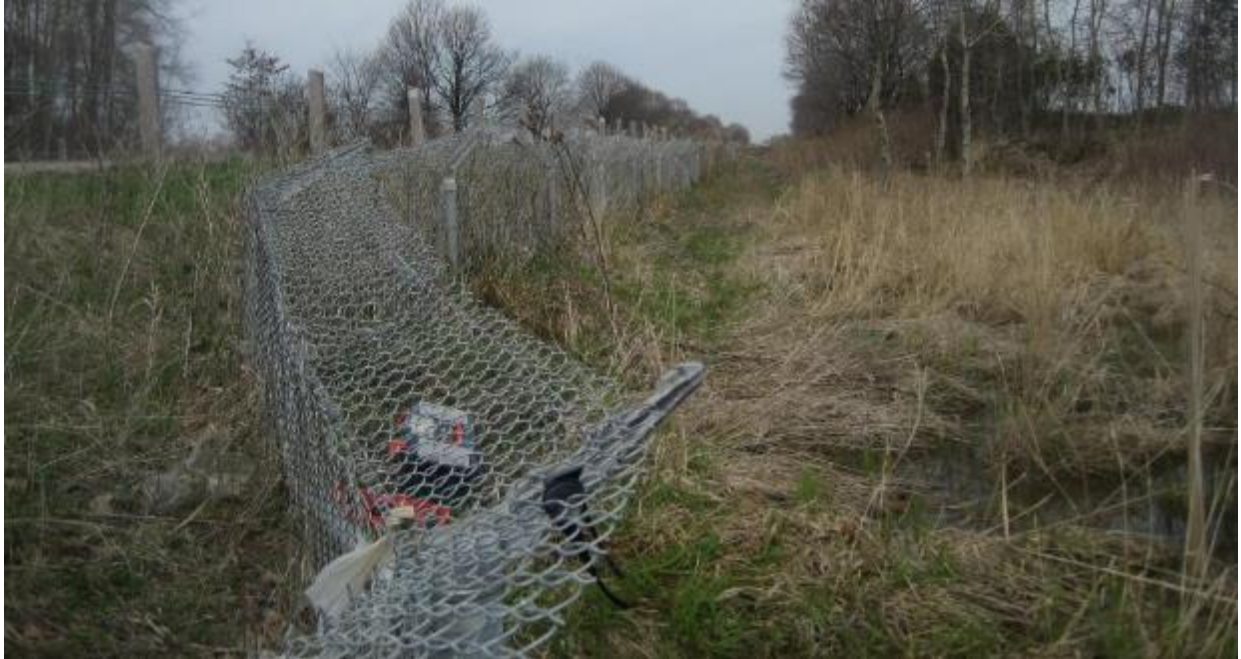
Figure 1: Top lip made from chain link fence and metal outriggers from top of fence. Photo Credit: Kari Gunson.
