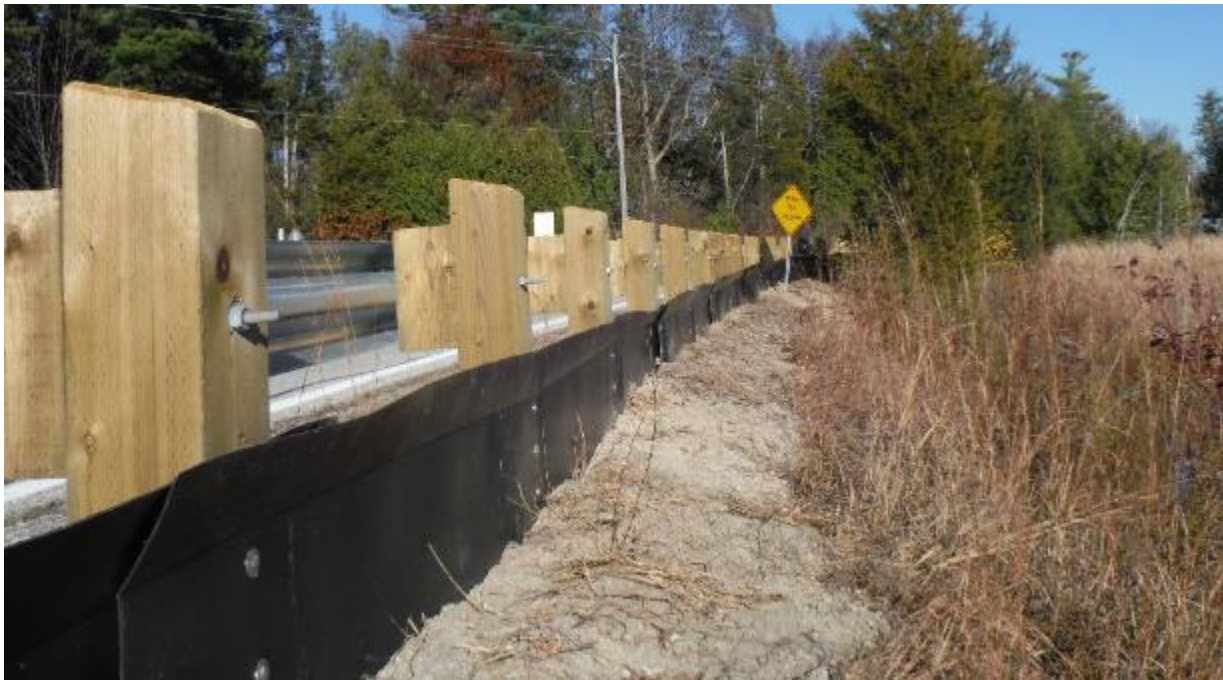
Figure 2: Plastic solid Animex fence with top lip and smooth surface to prevent climbing. Photo Credit: Ausable Bayfield Conservation Authority.
