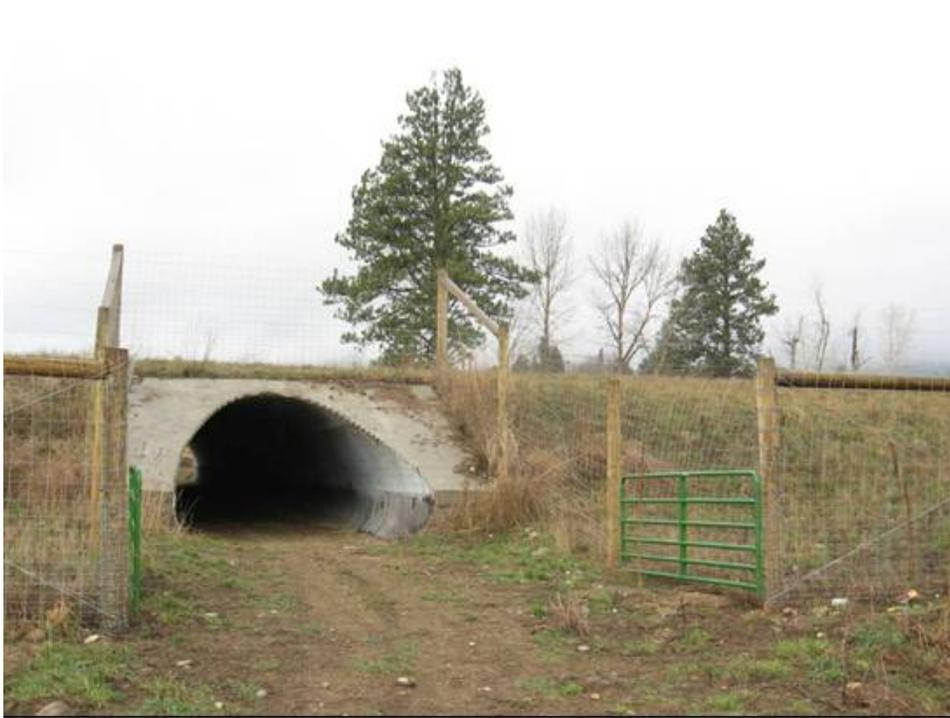
**Figure 80. An underpass designed for wildlife and human access, farm machinery and livestock along U.S. Highway 93, south of Missoula, MT (copyright: Marcel Huijser).**
