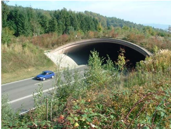
**Figure 60. A wildlife overpass in Germany. The terrestrial habitat connected by the overpass is at a higher elevation than the roadway (copyright: Mary Gray, FHWA).**
