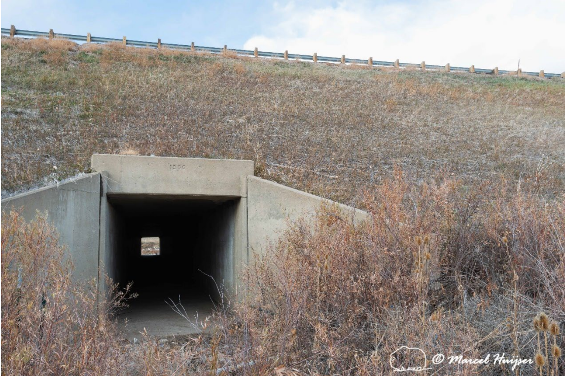
Figure 25: Surroundings, Rock Creek (Hwy 128, mile reference post 2.54), south side, inflow.
