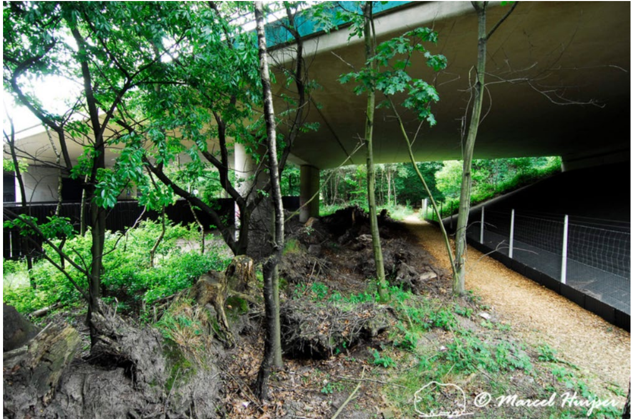
Figure 50. Multifunctional underpass under A28 motorway near Hilversum, The Netherlands. The trail for non-motorized human use is on the far-right side. A berm with root wads, small trees and shrubs in the center separates the trail from the wildlife zone further to the left. Beyond the black screen on the far left there is a 2-lane road.
