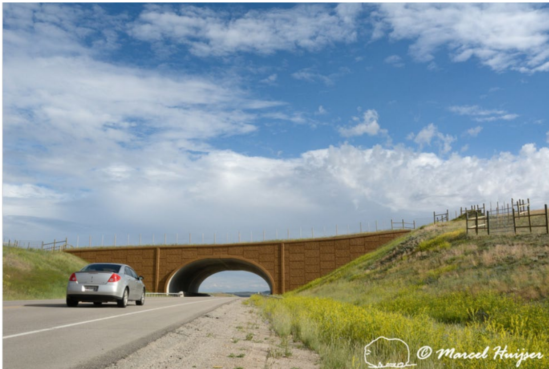
Figure 45. Wildlife overpass, primarily for pronghorn ( Antilocapra americana ) (46 m (150 ft) wide), on the Path of the Pronghorn, Trapper's Point, US Hwy 191, near Pinedale, Wyoming, USA.
