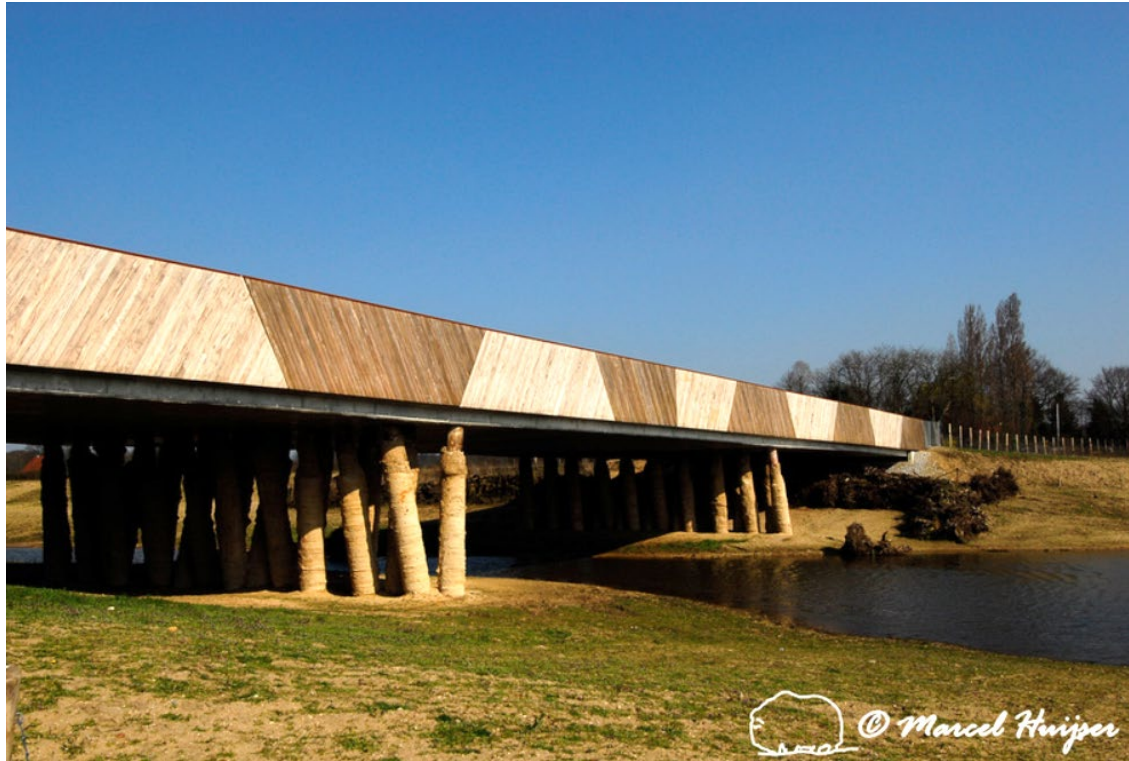
Figure 43. Multifunctional underpass, The Netherlands. The underpass is for hydrology and wildlife.
