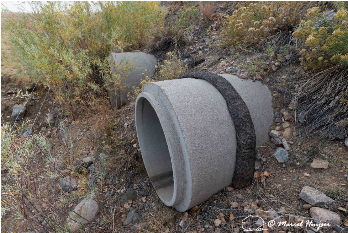
Figure 18: Double culvert, Woman Creek (Hwy 93, mile reference post 8.40), east side, outflow.
