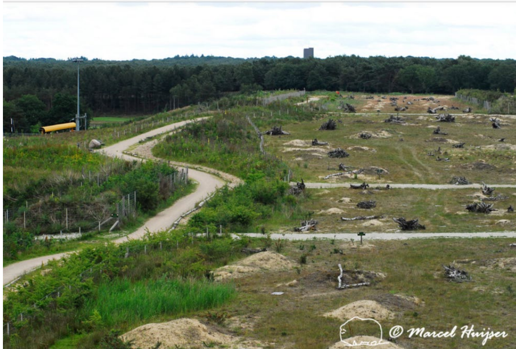
Figure 51. Multifunctional overpass across a 2-lane road and railroad tracks with a trail for non-motorized recreation on the left side, Natuurbrug Zanderij Crailoo, The Netherlands. The trail has a berm with trees and shrubs to reduce human presence and disturbance in the wildlife zone that is further to the right. The habitat on top of the overpass is dry and sandy grassland and heathland.
