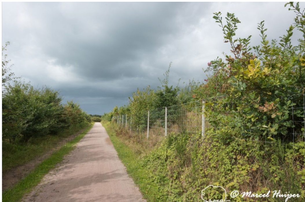
Figure 52. Multifunctional overpass across a 2-lane road and railroad tracks with a trail for non-motorized recreation, Natuurbrug Zanderij Crailoo, The Netherlands. The trail has a berm with trees and shrubs on the left-hand side to reduce human presence and disturbance in the wildlife zone that is further to the left. There is also a berm with trees and shrubs to the right of the trail, reducing visual and noise disturbance from vehicles towards the trail.
