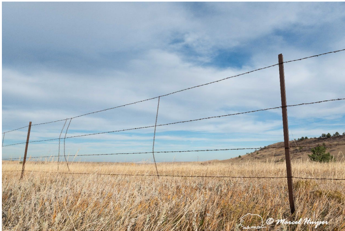
Figure 34: Right-of-way fence, Hwy 93, east side, near mile reference post 11.3.
