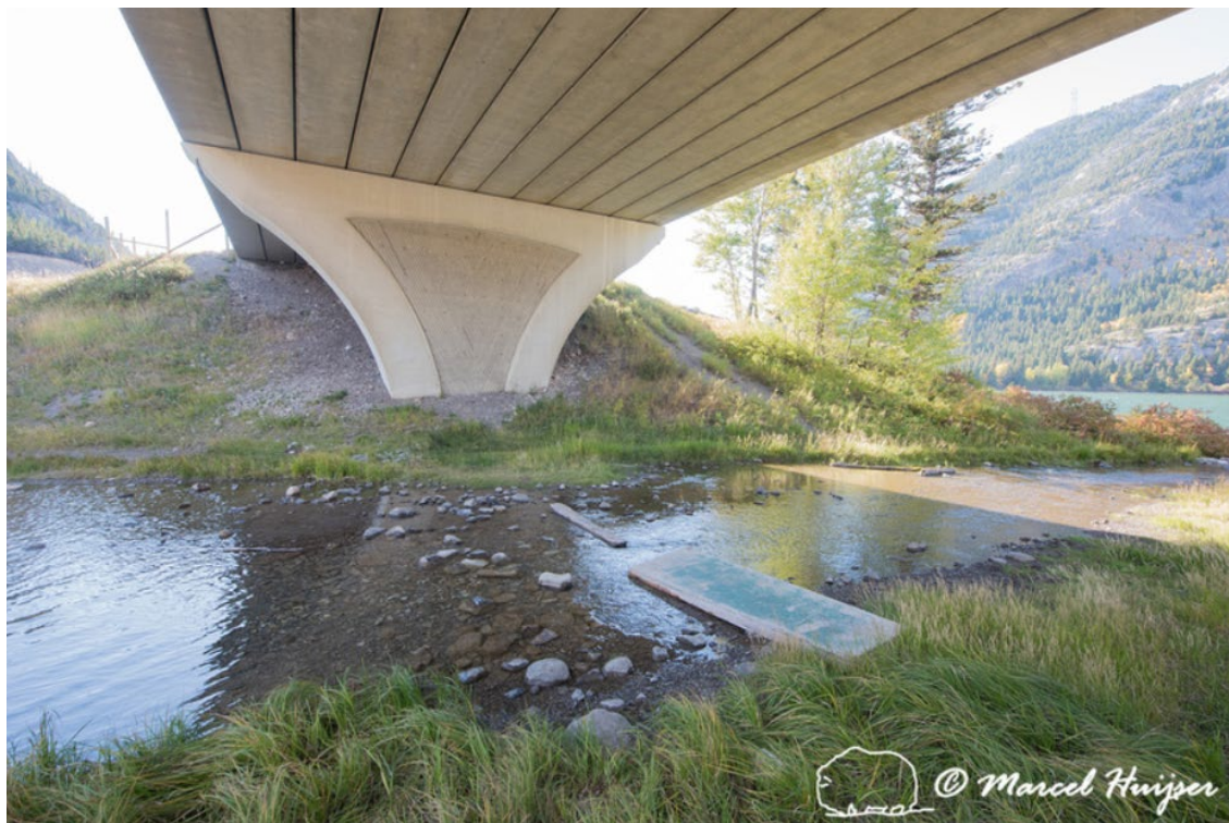
Figure 44. Multifunctional underpass, Hwy 3, Crowsnest Pass, Alberta, Canada. The underpass is for hydrology and wildlife. Note how the substrate and stream dynamics are unaffected by the structure and how light and moisture reaches the entire area under the bridge allowing for natural vegetation in the riparian and terrestrial zones.
