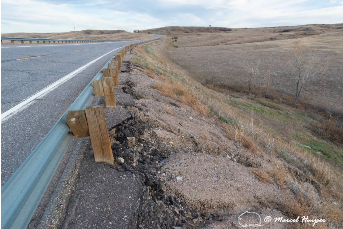
Figure 24: Surroundings, Rock Creek (Hwy 128, mile reference post 2.54), south side, looking east.
