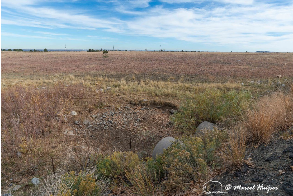
Figure 17: Double culvert, Woman Creek (Hwy 93, mile reference post 8.40), east side, outflow.
