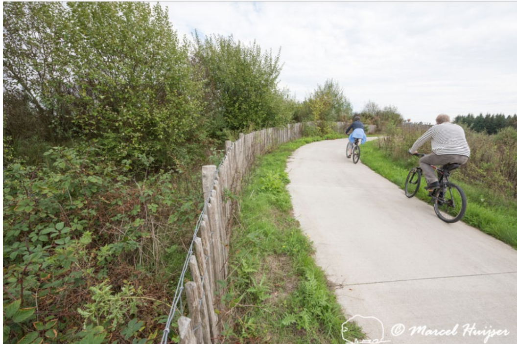
Figure 54. Bicyclists on a trail on a multifunctional overpass. The trail is for non-motorized recreation. Soest, The Netherlands. The trail has a fence and a berm with trees and shrubs on the left-hand side to reduce human presence and disturbance in the wildlife zone that is further to the left.
