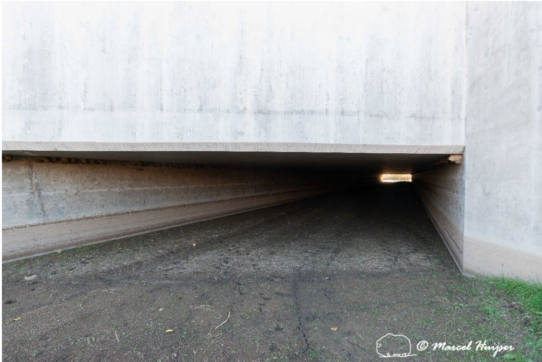
Figure 38: Culvert at Davidson Ditch (Hwy 36, mile reference post 40.8).
