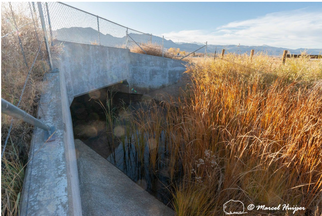
Figure 39: Culvert at Goodhue Ditch (Hwy 36, mile reference post 41.2).
