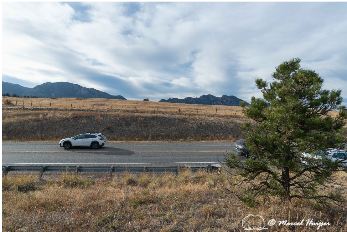
Figure 46. The roadcut along Hwy 93, around mile reference post 11.3.
