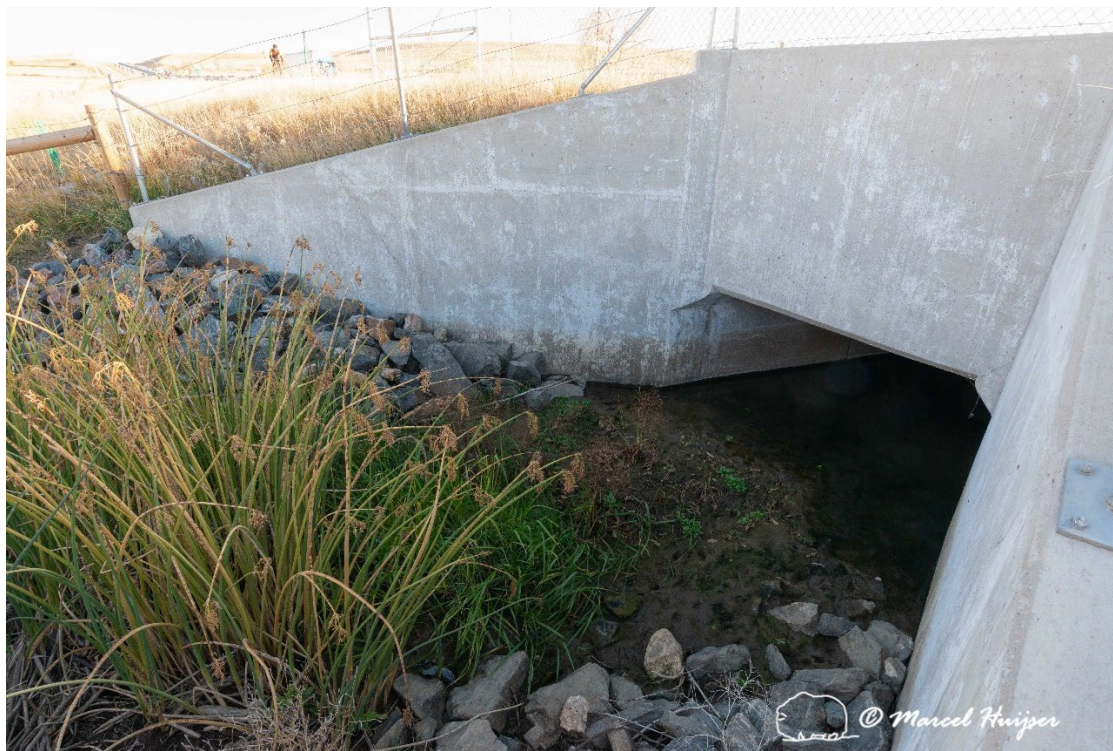
Figure 40: Culvert at Marshallville Ditch (Hwy 36, mile reference post 41.5).
