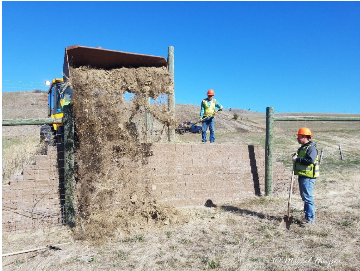
Figure 4: The Montana Department of Transportation assisted with the lowering of 10 jump-outs. After removing concrete blocks of the face, soil from the top was deposited at the bottom for the landing area.
