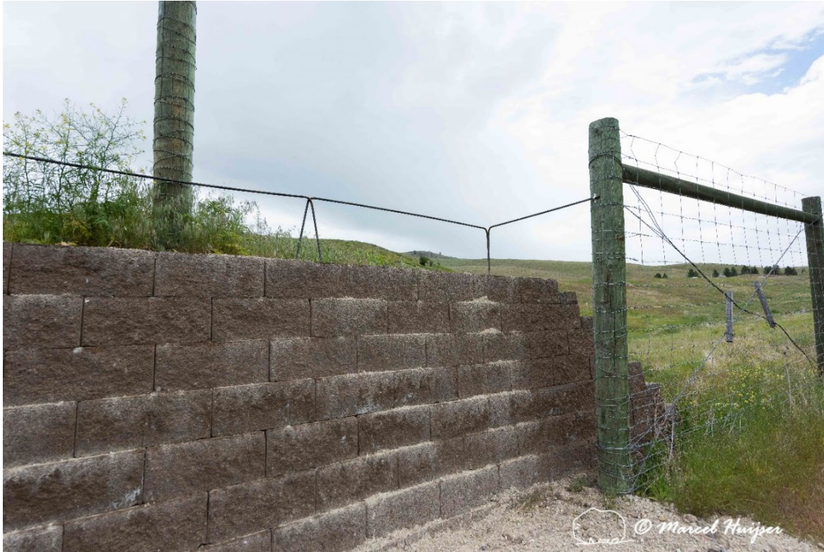
Figure 7: The rebar installed with the L-shaped corner elements connected to the fence post.
