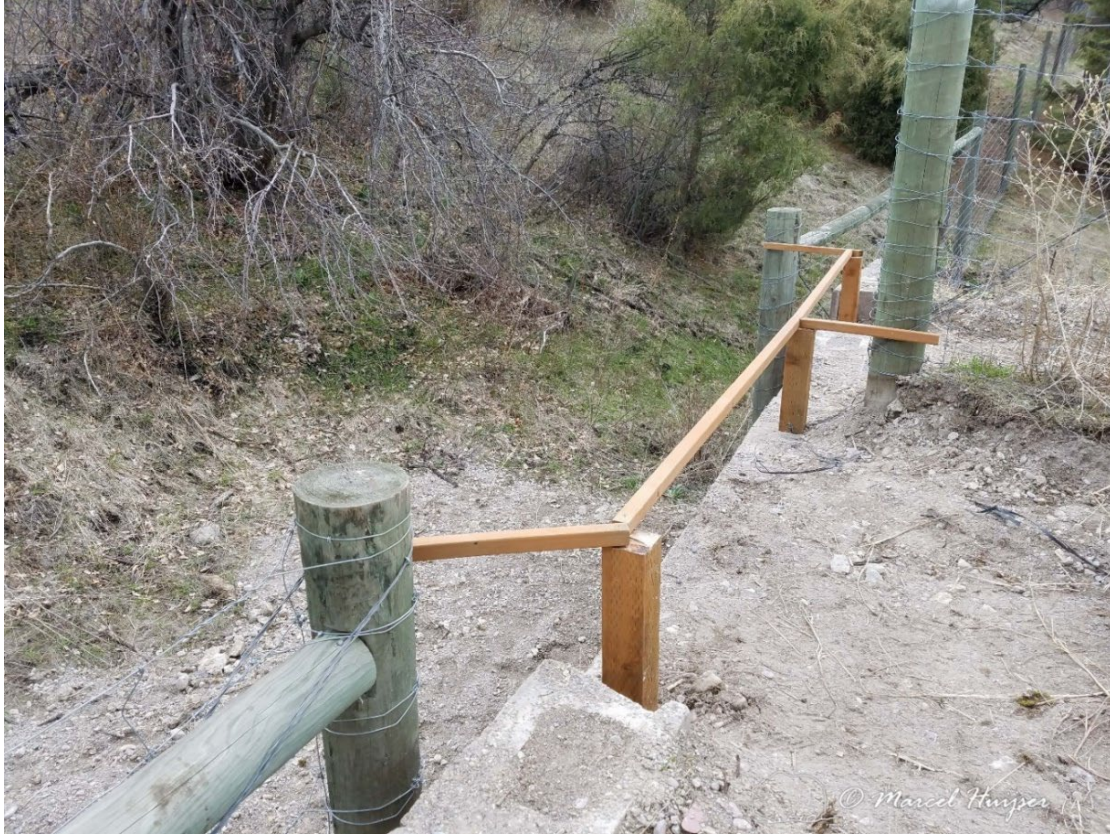
Figure 5: The prototype for the “bar” made from “5x5” cm (“2x2” inch) and “10x10” (“4x4” inch) treated lumber.
