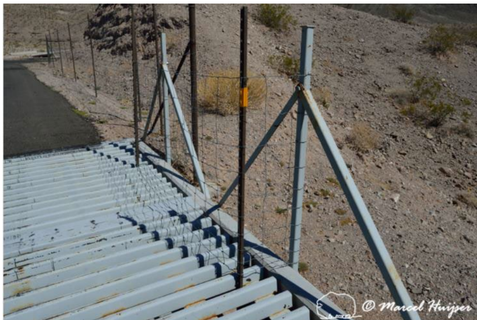
Figure 17. Blocked concrete edge at side of wildlife guard at access road US Hwy 93, Arizona, USA. Some wildlife species will walk on the narrow concrete edge of the wildlife guard to access the fenced road corridor. The concrete edge is part of a wall for the pit under the metal bars. Here the edge is made inaccessible to large mammals through an extra piece of wildlife fence.
