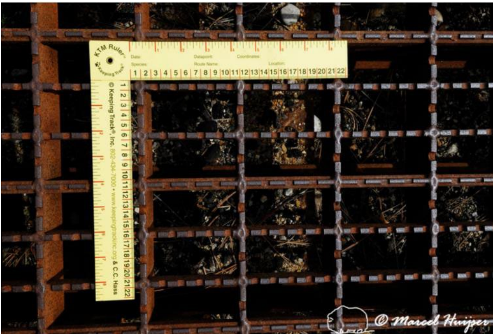
Figure 21. Detail of the modified bridge grate material used for wildlife guards installed at access roads along US Hwy 93, near Ravalli, Montana, USA. This material is more suitable for pedestrians and cyclists compared to the bars of a traditional wildlife guard or cattle guard.
