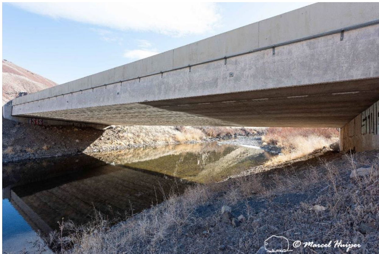
Figure 49. An open structure with a clear line-of-sight towards the other side of the road is recommended. Note that this structure would still benefit from a dry flat path with sand or gravel.
