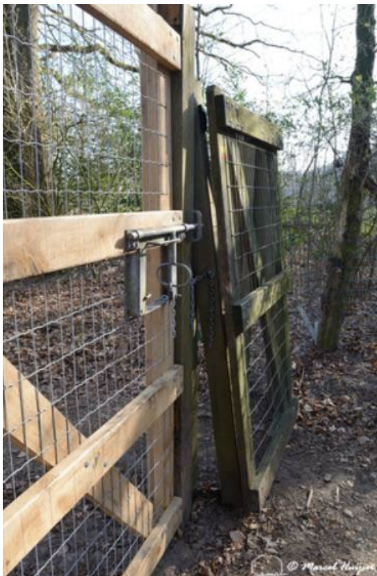
Figure 23. Swing gate at a wildlife fence, set at an angle so it closes through gravity, The Netherlands.
