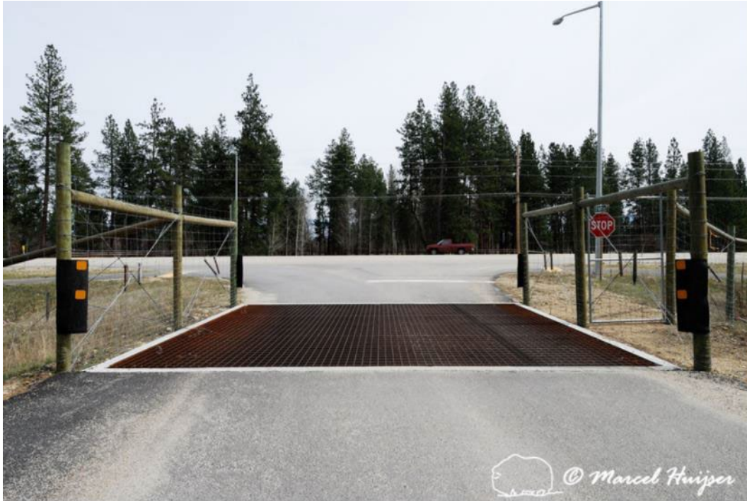
Figure 14. Wildlife guard installed at an access road to the main highway (US Hwy 93S), near Stevensville, Montana, USA. The metal barrier is easy to walk and bike over. Note that the concrete ledge can be used by wildlife to access the fenced road corridor. This concrete ledge should be made inaccessible.
