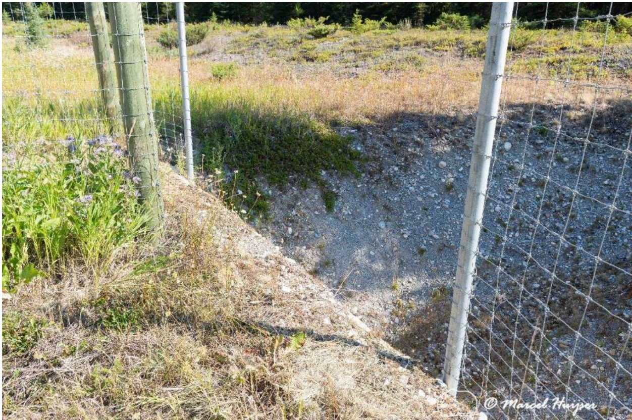
Figure 32. Wildlife fence with jump-out, Kootenai National Park, British Columbia, Canada. The pit is dug on the habitat side of the fence.
