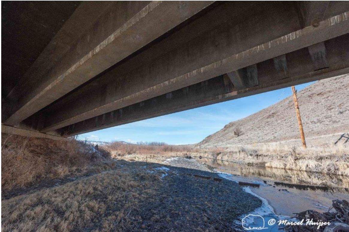
Figure 41. This bridge is sufficiently wide and high for mule deer, it has a good line-of-sight through the structure, and there is enough dry and flat terrain for them to travel under the bridge, at least in winter.
