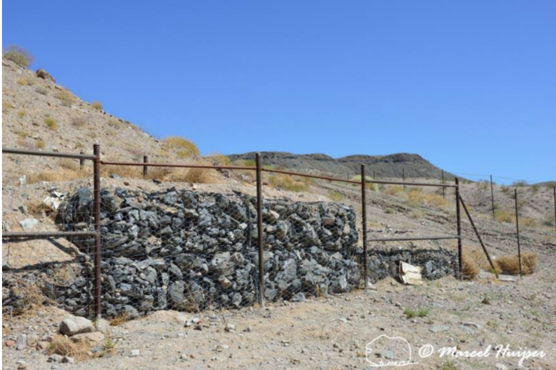
Figure 26. Wildlife jump-out or escape ramp with a rock wall and bar designed for desert bighorn sheep ( Ovis canadensis nelsoni ), US Hwy 93, Arizona, USA. The bar reduces the probability that bighorn sheep will jump up into the fenced road corridor while it does not decrease the probability that the bighorn sheep will jump down to the safe side of the fence. The sheep can crawl under the bar before jumping down.
