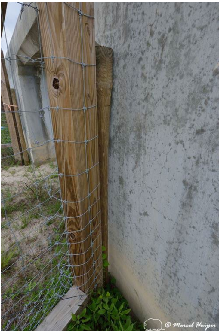
Figure 6. Tight connection (no gap) between last fence post and wall of the wildlife underpass, Hwy 331, Hwy 83 near Freeport, Florida, USA. The angle at which the fence comes in does not result in a dangerous wedge or funnel that could lead to animals getting trapped.
