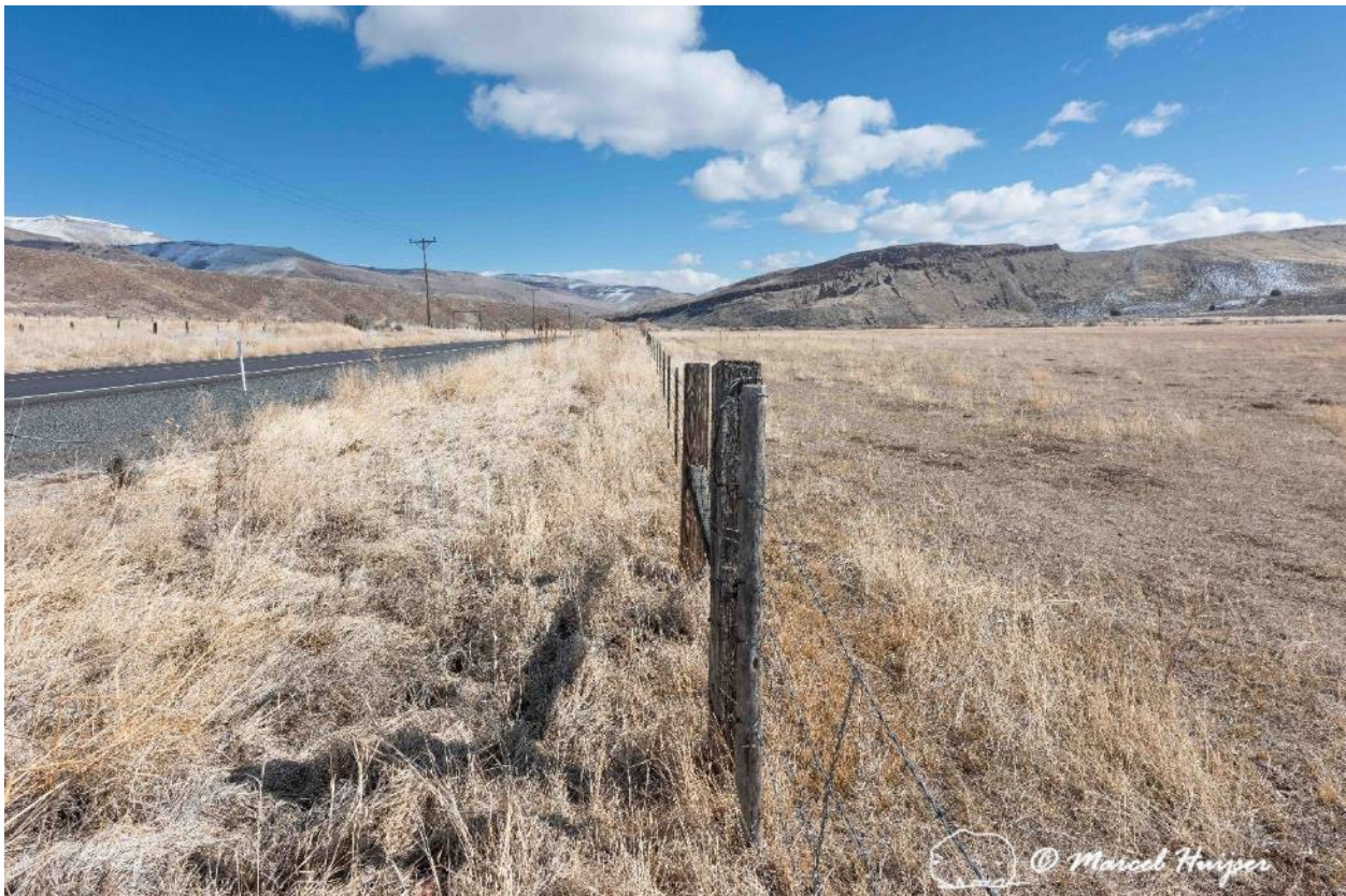
Figure 39. Right-of-way or livestock fence along US Hwy 20 between Juntura and Harper, Oregon.
