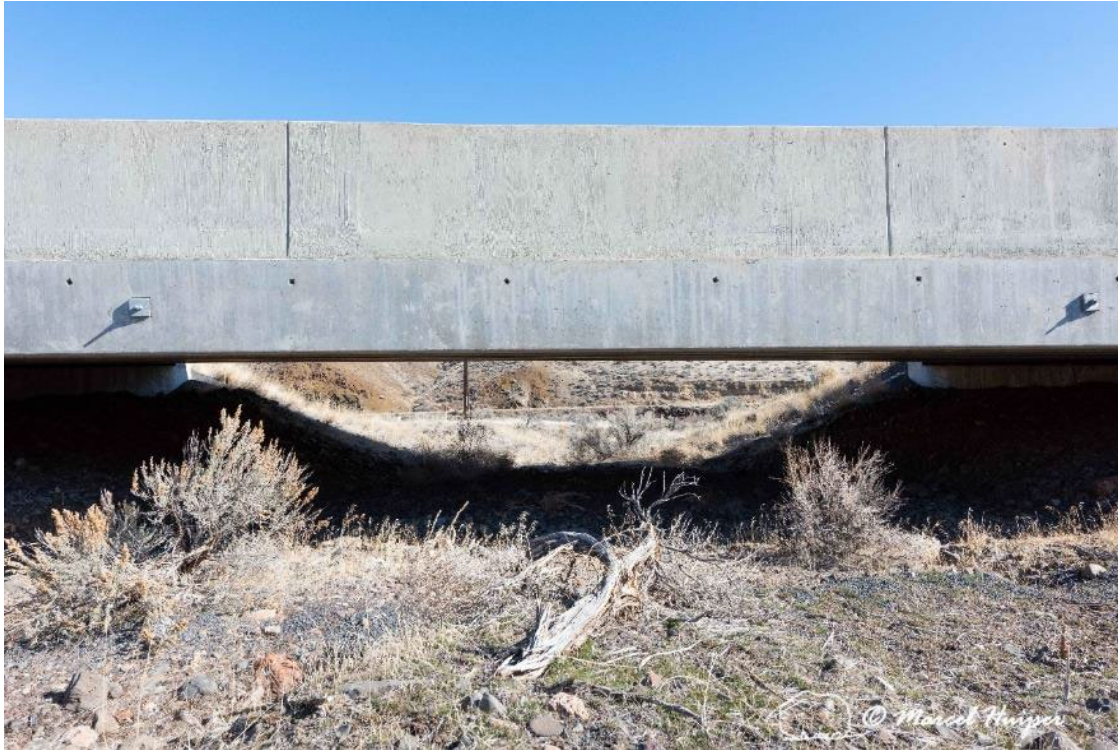
Figure 45. Low clearance (height) of a structure likely impacts use by large wild mammals, including deer.
