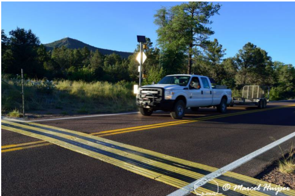
Figure 12. Electrified mat associated with an animal detection and driver warning system at a fence-end, S.R. 260 east of Payson, Arizona, USA.
