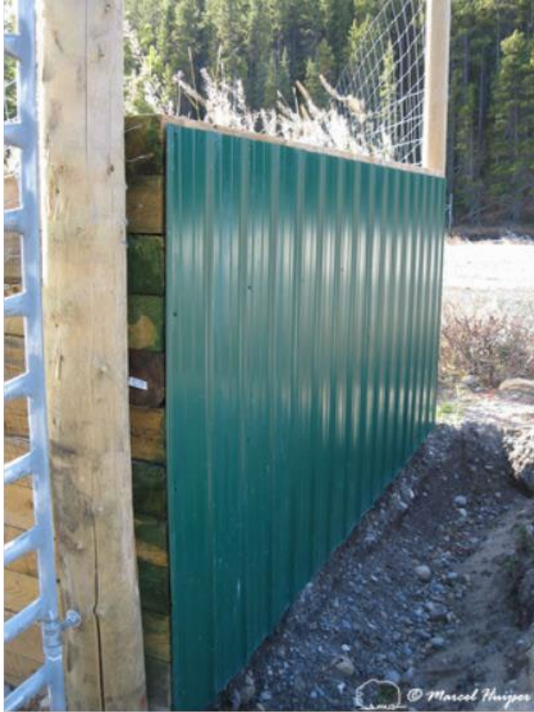
Figure 29. Wildlife jump-out with a smooth metal face to reduce the likelihood that bear will climb the jump-out and end up in fenced right-of-way, Banff National Park, Alberta, Canada.
