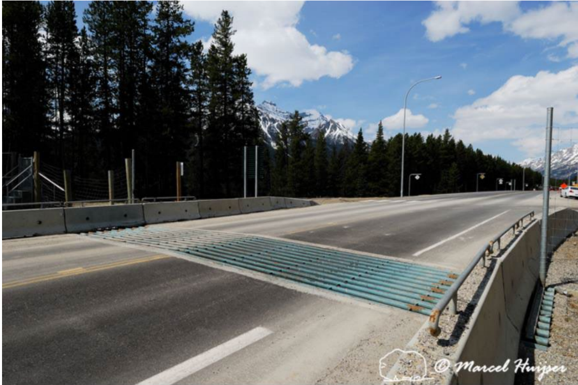
Figure 9. Fence-end brought close to the edge of the pavement, protected by Jersey barriers. Also note that there is a wildlife guard embedded in the travel lanes, Alberta, Canada.
