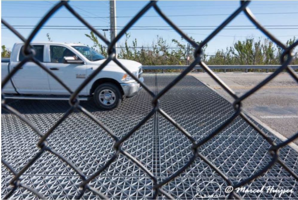
Figure 11. Wildlife guard at a fence-end on US Hwy 1, Big Pine Key, Florida, USA.
