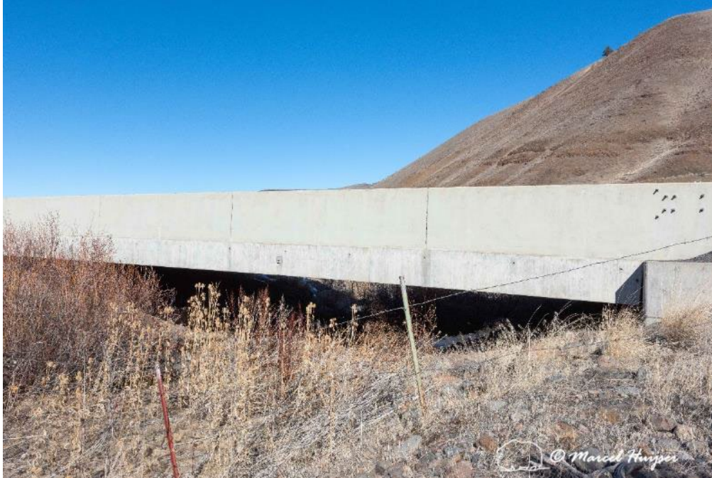
Figure 43. A right-of-way or livestock fence hinders access to the structure for large wild mammals. If this fence is still needed, consider replacing it with a wildlife friendly livestock fence.
