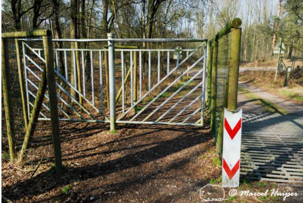
Figure 24. Wildlife guard (right) and horse gate (left), Heugterdijk, Weerterbos, near Maarheeze, The Netherlands. The riders do not have to dismount and can push the rotating gate while in the saddle. The gate is set at an angle so that gravity will bring the rotating fence in line with the main fence.
