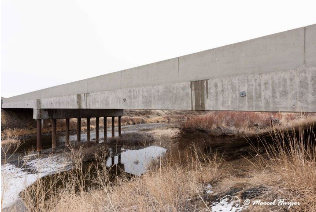
Figure 50. A structure with pillars can still allow for visibility under the bridge and a good line-of-sight towards the other side of the road. Note that this structure would still benefit from a dry flat path with sand or gravel with sufficient clearance (height).
