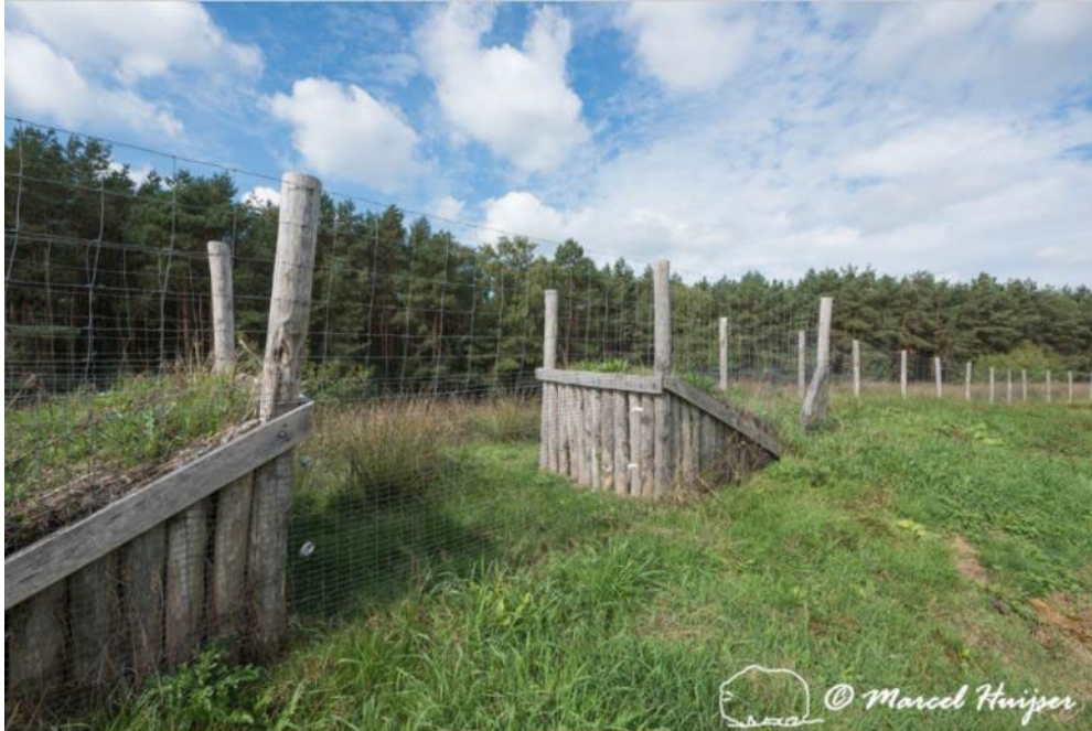
Figure 31. Wildlife fence and jump-out along A28 motorway, near Spier, Drenthe, The Netherlands. The fence is a barrier for medium and large mammal species. The electric fence is an additional barrier for livestock (sheep, cattle) that are used as a tool for nature management in the area.
