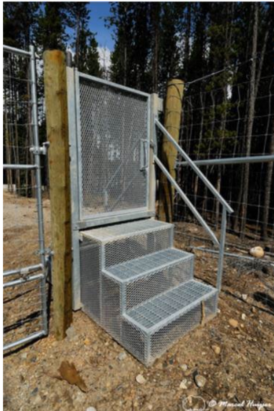
Figure 25. Pedestrian gate with steps (for high snow accumulation) at a wildlife fence, Alberta, Canada.
