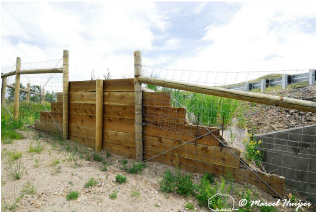
Figure 30. Wildlife fence and jump-out with a face consisting of wooden planks, near Havre, Montana, USA.
