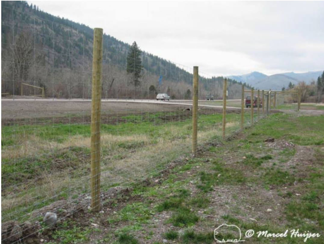
Figure 5. Typical large ungulate fence in North America, 8 ft tall, wooden posts and mesh-wire fence material, US Hwy 93 North, Montana, USA. Note that there is a dig barrier attached to the main fence material (e.g. for canids).
