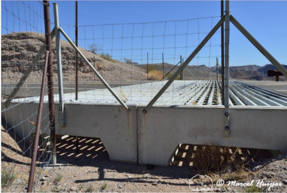
Figure 18. Combined drainage and escape for small animals under wildlife guard, Arizona, USA. The openings on the side allow for drainage under the culvert. The openings also allow invertebrates, amphibians, reptiles, small mammals and other species that may fall in between the metal bars to escape.
