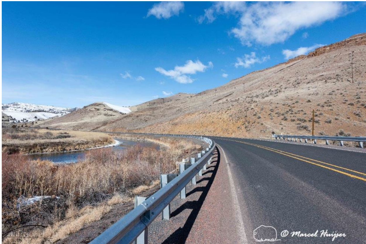
Figure 40. There is little space for a wildlife fence between the Malheur River and US Hwy 20, and floods may jeopardize the stability of the fence.
