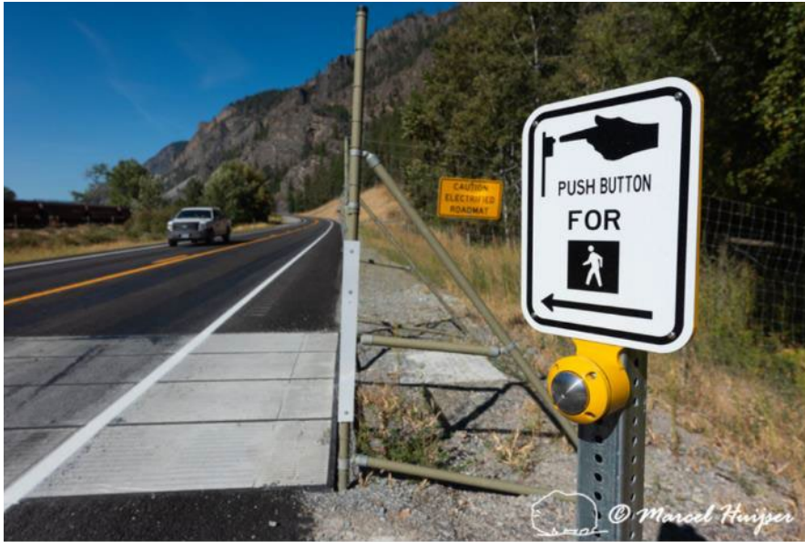
Figure 22. Push button on timer (turns electricity off for 1 minute) for pedestrians at an electrified barrier embedded in travel lanes to keep large mammals, including bighorn sheep, out of fenced road corridor, MT Hwy 200, Thompson Falls, Montana, USA.
