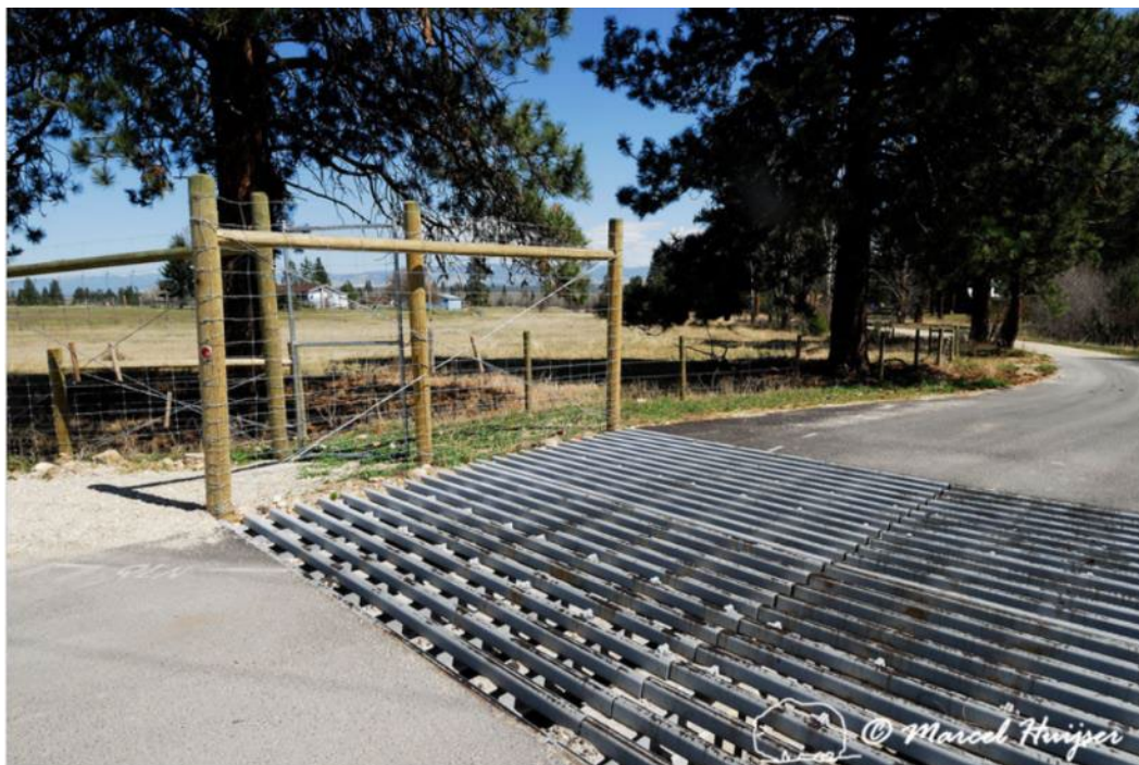
Figure 15. Wildlife guard at an access road to US Hwy 93S, near Victor, Montana, USA. This type of wildlife guard is less suited for pedestrians and cyclists.
