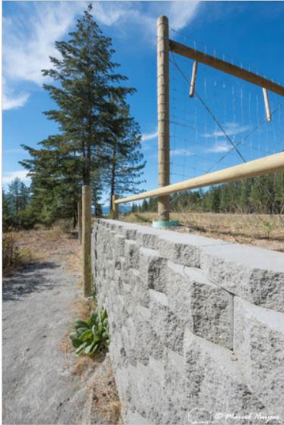
Figure 27. Wildlife jump-out with concrete blocks and a bar for bighorn sheep ( Ovis canadensis ), near Thompson Falls, Montana, USA. Note that it is probably better to not have the concrete blocks protrude as it makes it easier for species to climb the face.
