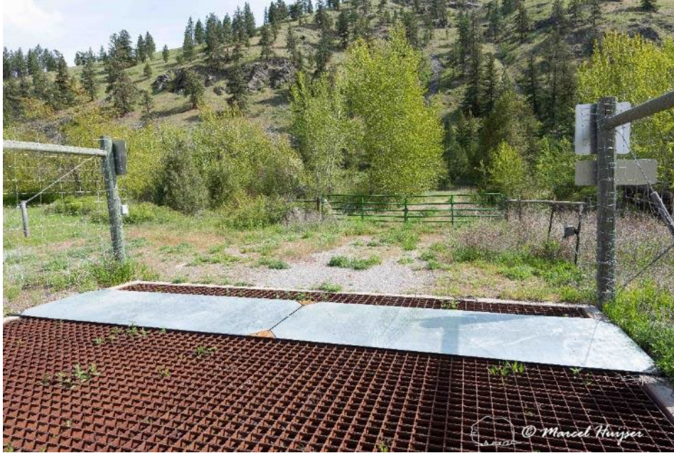
Figure 16. Electrified barrier, designed for low traffic volume and low traffic speed, on top of a wildlife guard at an access road to US Hwy 93S, near Ravalli, Montana, USA.
