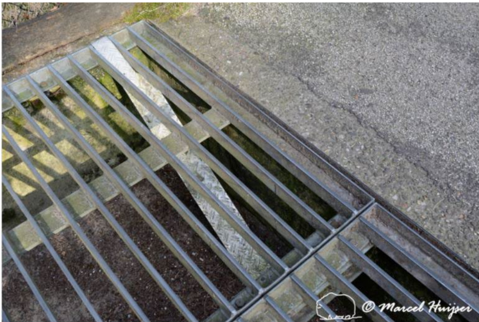
Figure 19. For wildlife guards that have a fully enclosed pit with contiguous walls sometimes wooden planks or metal strips are attached, potentially allowing small animal species to climb out of the pit.
