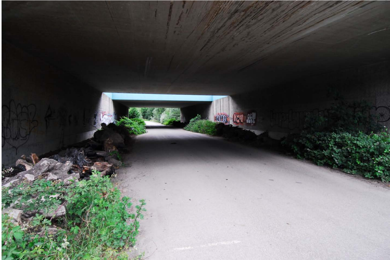
Figure 3.1: A row of tree stumps provides cover for invertebrates, amphibians, reptiles, and small mammals inside a modified underpass originally build for traffic alone under a motorway (Copyright: Marcel Huijser). Note that vegetation grows where there is sufficient light and moisture, including in the median in between the two structures (one structure per travel direction).
