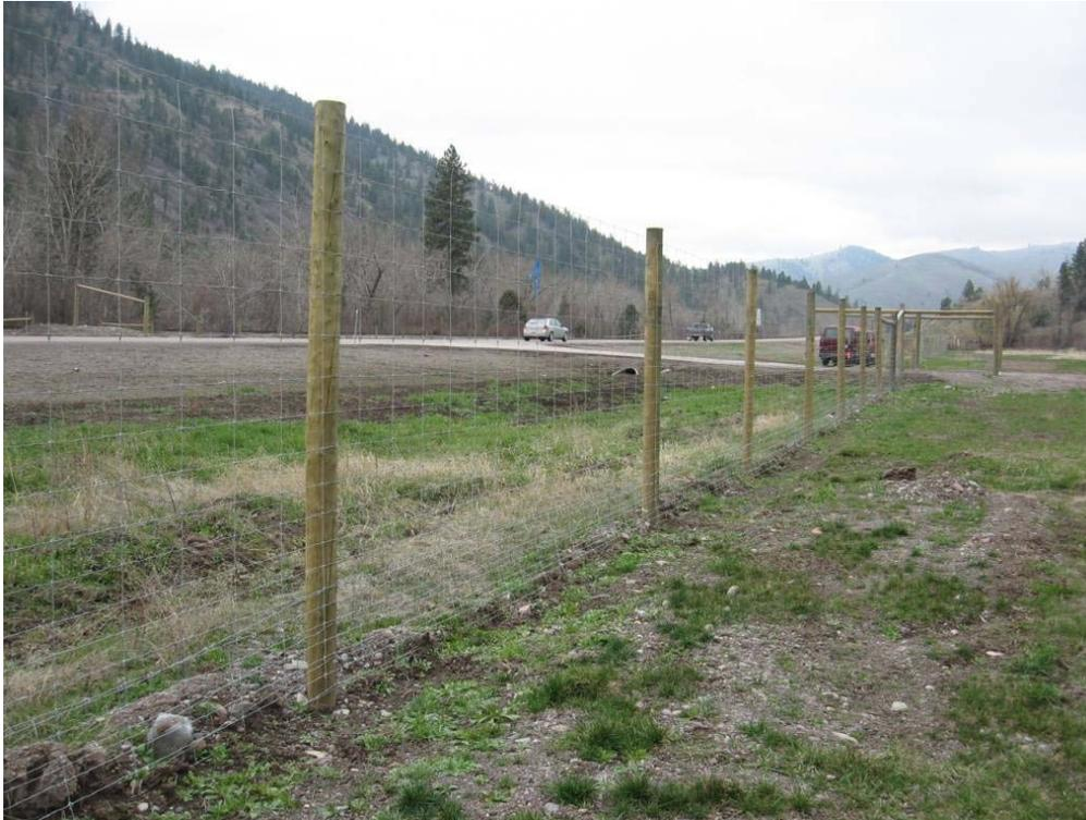
Figure 3. A wildlife fence (2.4 m (8 ft) high) designed to keep large ungulates from entering the road corridor (© Marcel Huijser).
